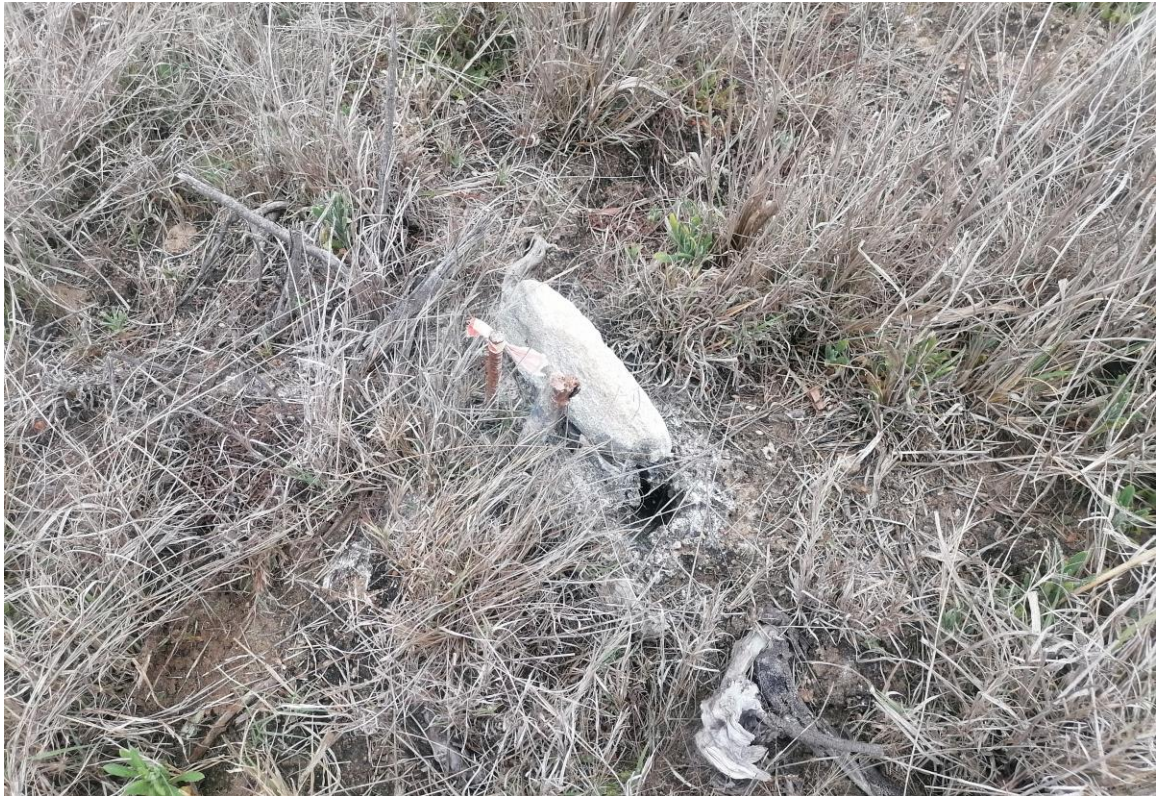
Photo 3: Show the peg on site, where the pole will be planted
