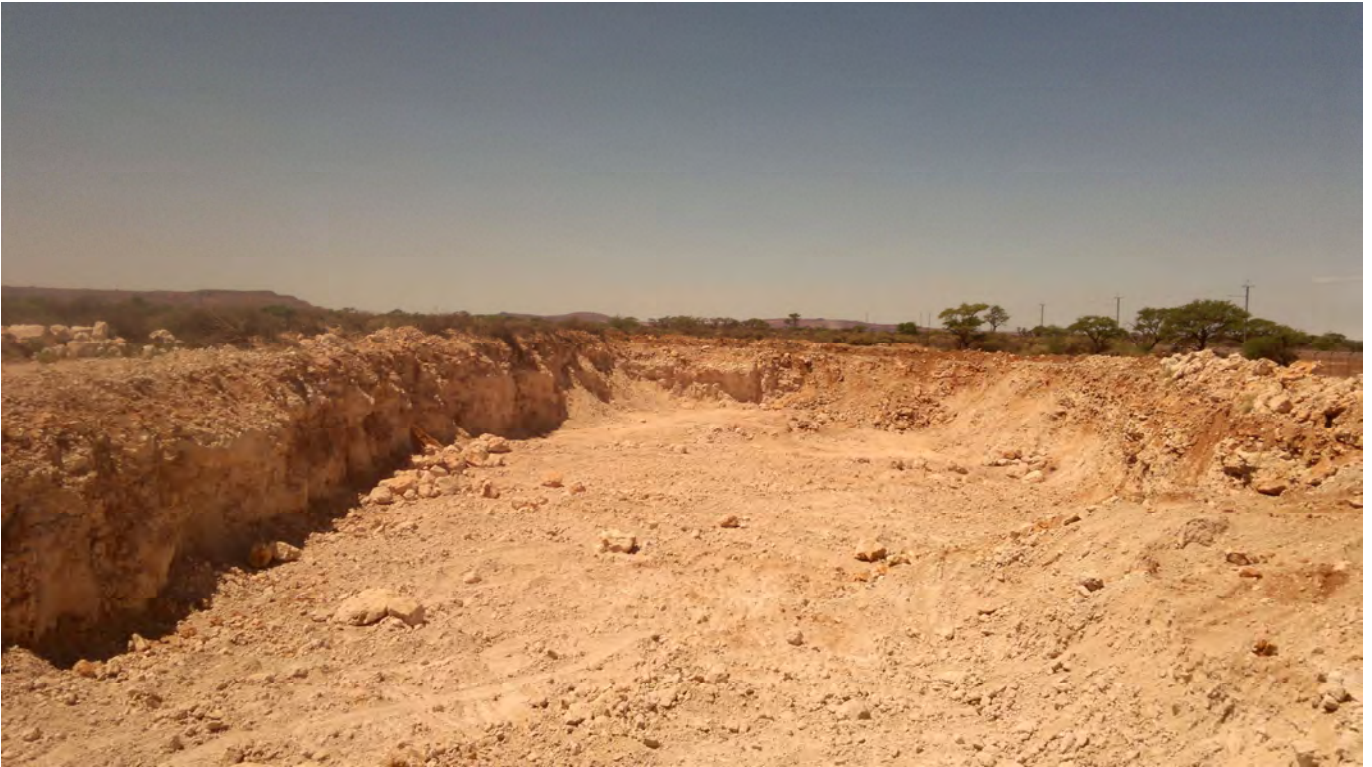
Plate 1: View to the South from the Northern side of the borrow pit
