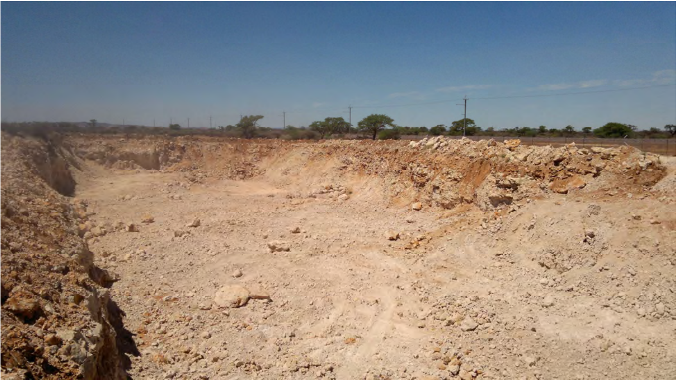
Plate 3: View to the South West from the Northern side of the borrow pit
