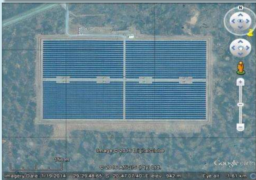
Photo and sat image of an existing PV project
