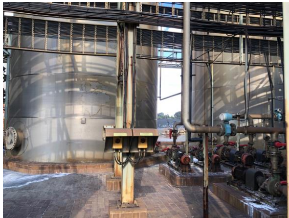
Existing barren treatment tanks which will be used as settling tanks
