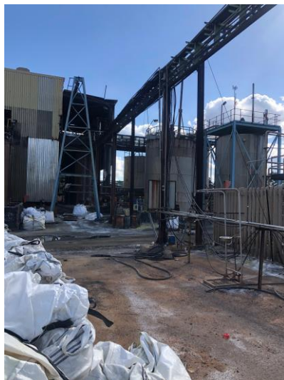
Looking from the proposed location (west) towards the Chemical Plant
