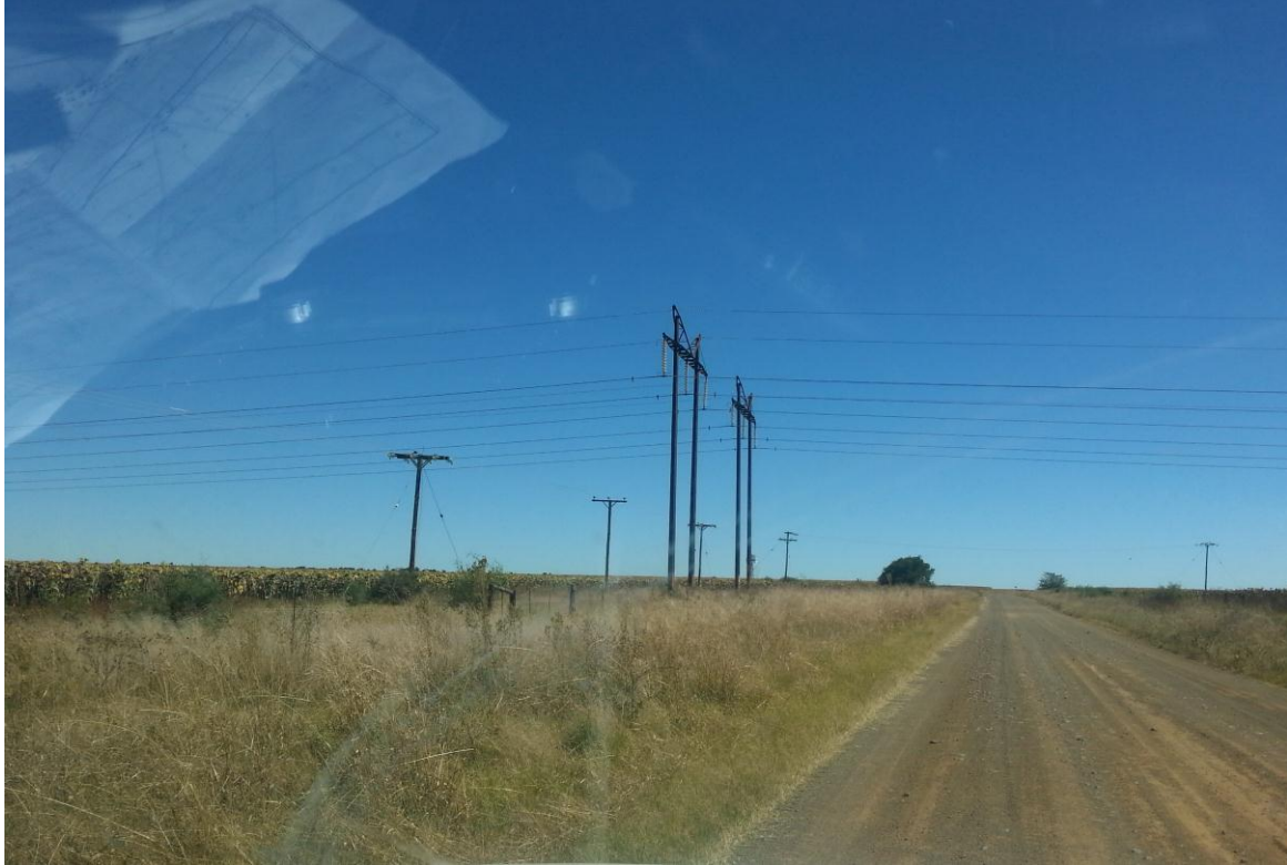
Image 15: Existing 132Kv line
