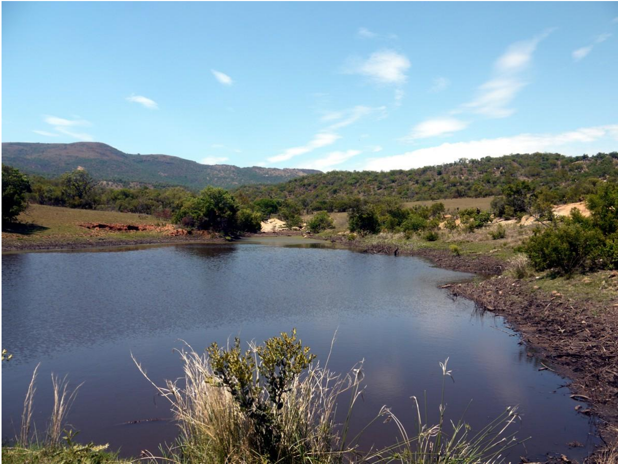
Plate 18, Sand Pile Dam, view looking south at the dam from the dam wall.
