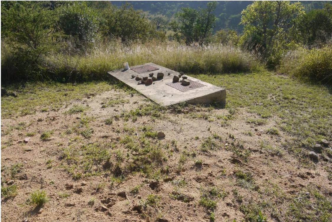
Plate 25, An existing soak pit that is currently used for disposal of sewage and grey water. This system is likely to be inadequate for the proposed reception facility
