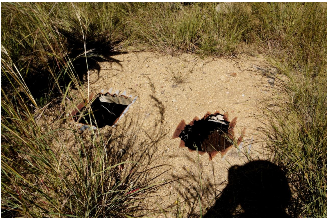
Plate 33, Leopard Rock, original soak away system.
