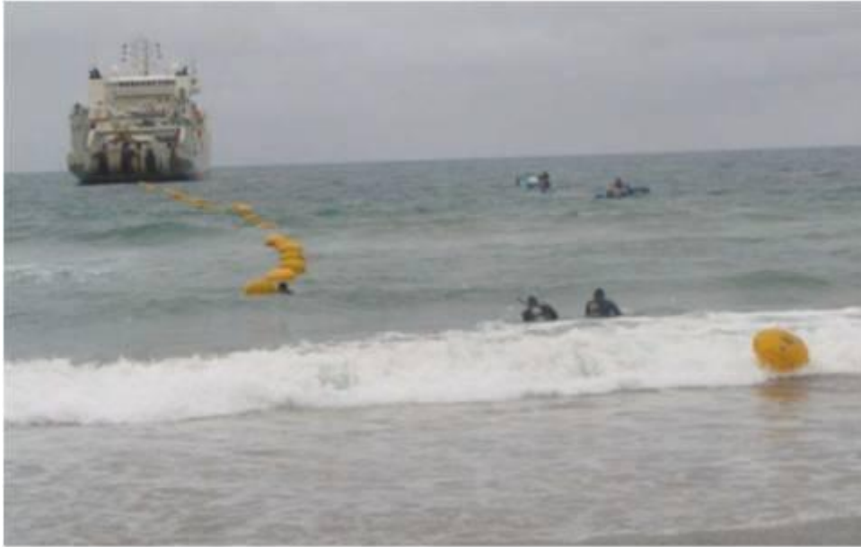
Figure 7 Cable being guided to shore by divers and small boats
