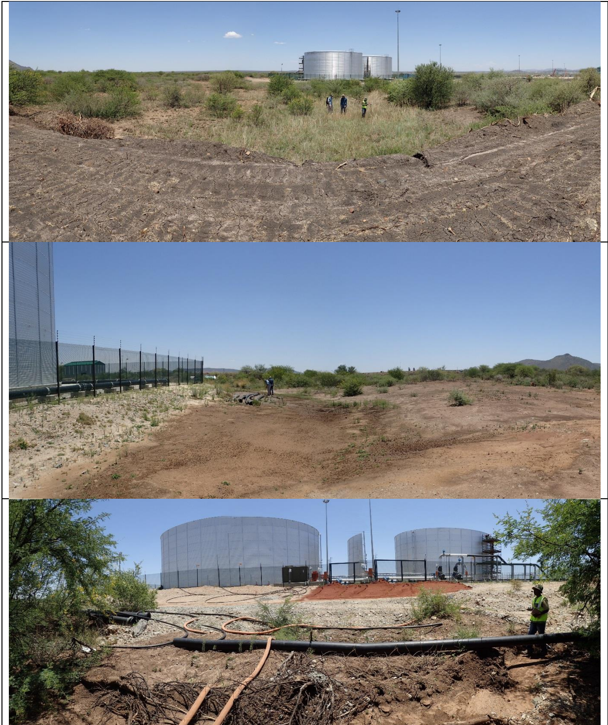
Figure 12: Illustrates existing impacts within Unchannelled valley bottom wetland 1 associated with existing mining infrastructure: A newly created 'noise berm' that bisects the wetland and prevents surface flow (top) (also refer to Figure 3 regarding existing infrastructure in the wetland); A diversion of the flow path of the wetland around steel tower infrastructure (centre) (also refer to Figure 3); & Channel development in the wetland downstream of the flow path diversion (bottom).
