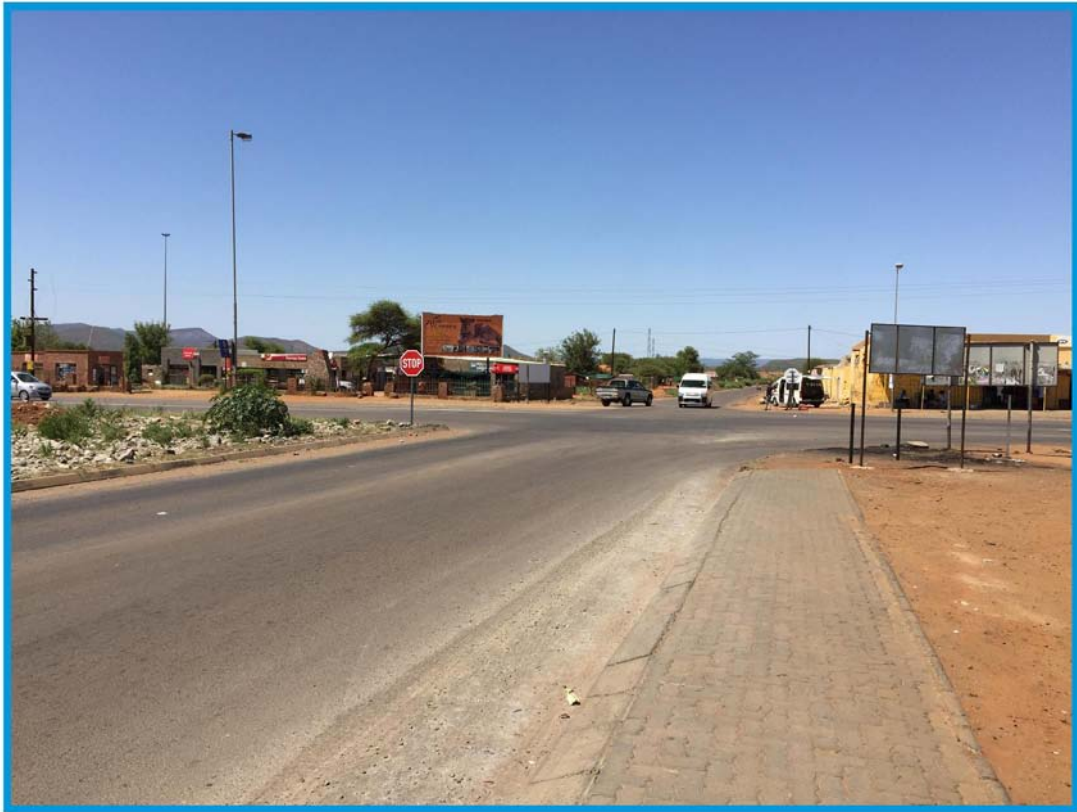
Photo 2: R556 East Approach
