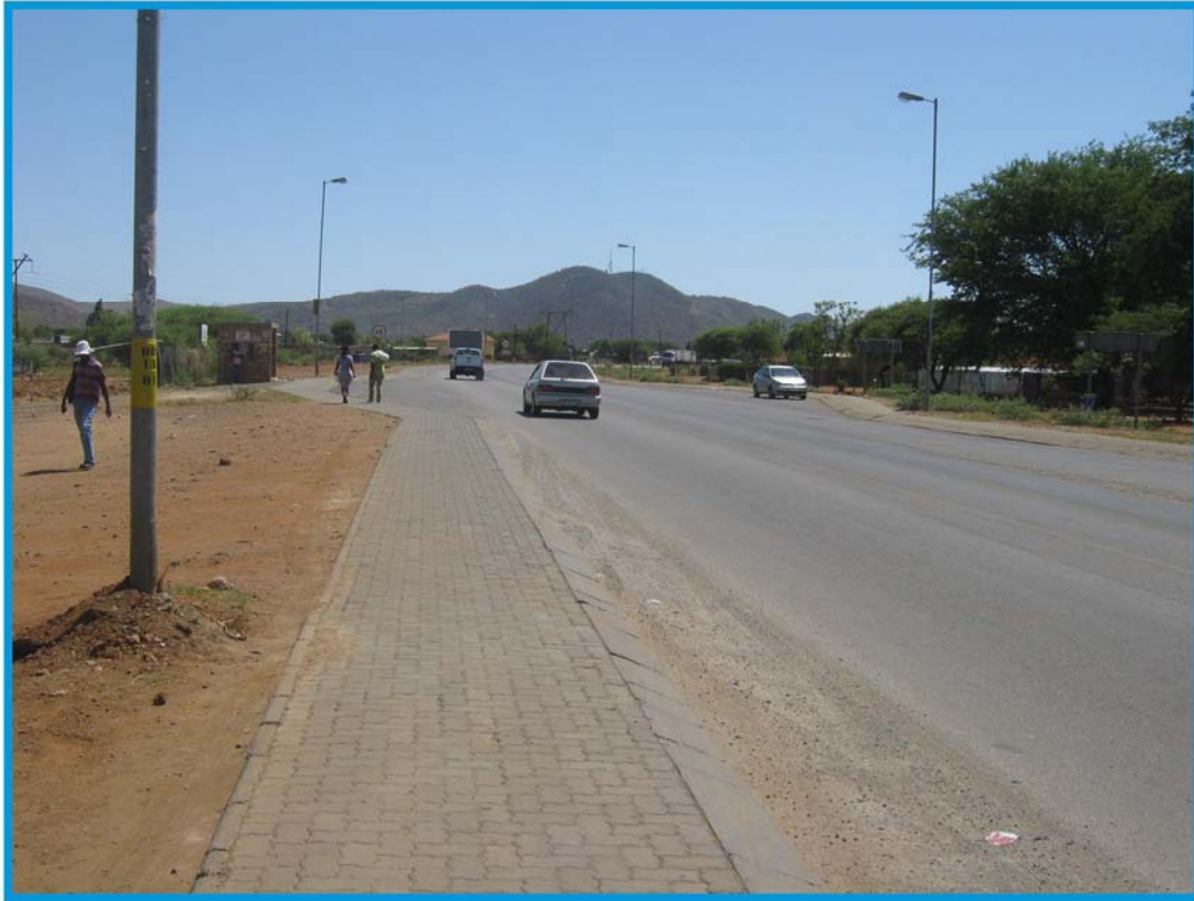
Photo 7: R556 East of R556 & R565 Intersection
