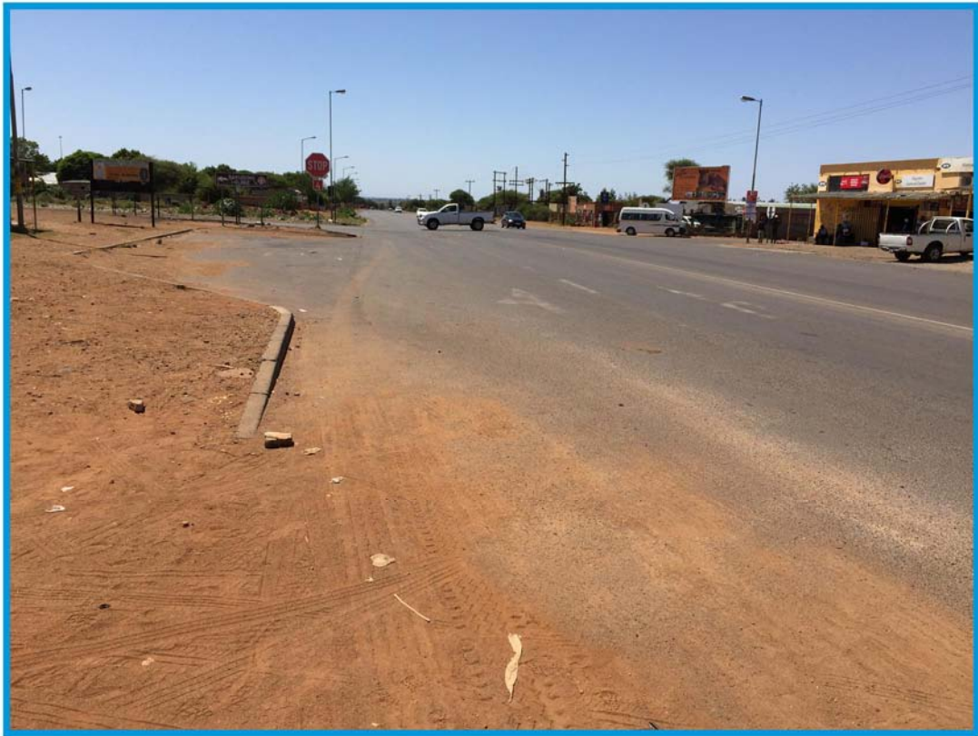
Photo 1: R565 North Approach
