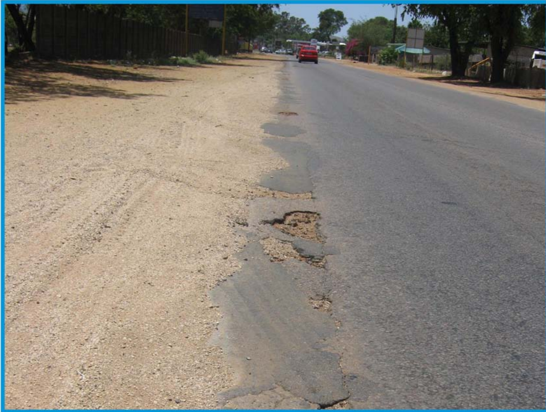
Photo 19: Edgebreaks along the R565, through Boshhoek
