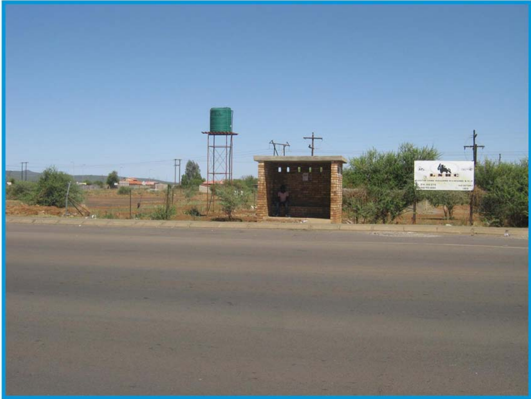
Photo 9: Bus Shelter along R556
