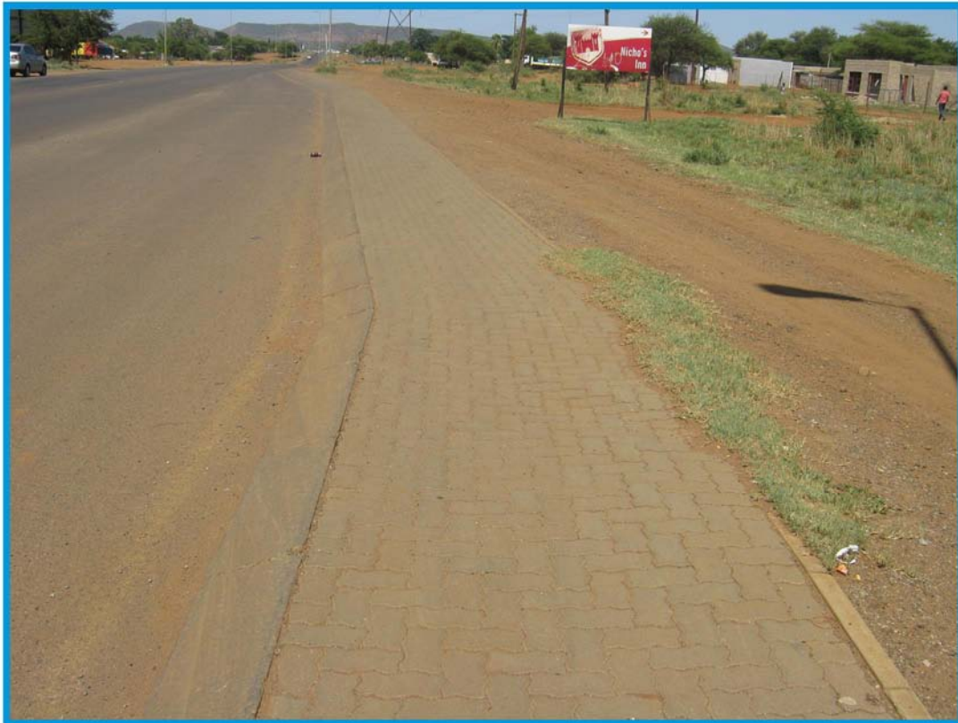
Photo 8: Public Transport Bay
