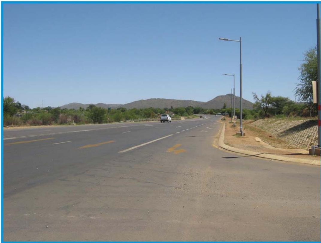
Photo 14: Sight Distance From Beyond Stop Line, North
