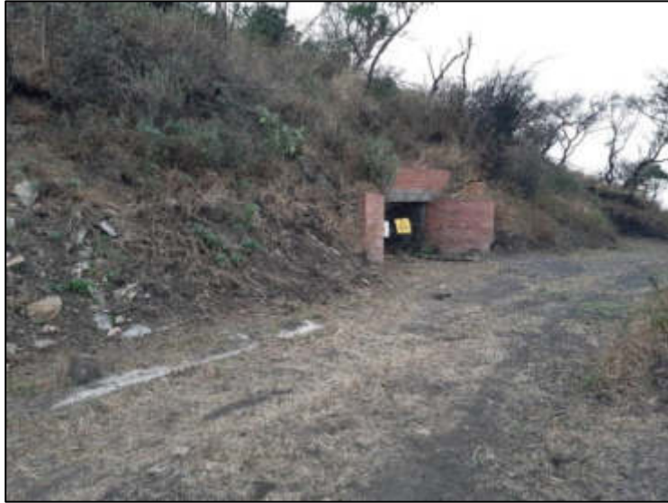
PLATE 3-1: EXISTING ADIT ON SITE
