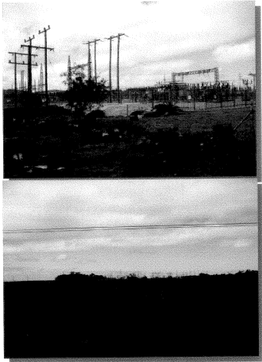
Figure 3.1: Melkhoutbosch substation, near the N2-R330 interchange north of Humansdorp
