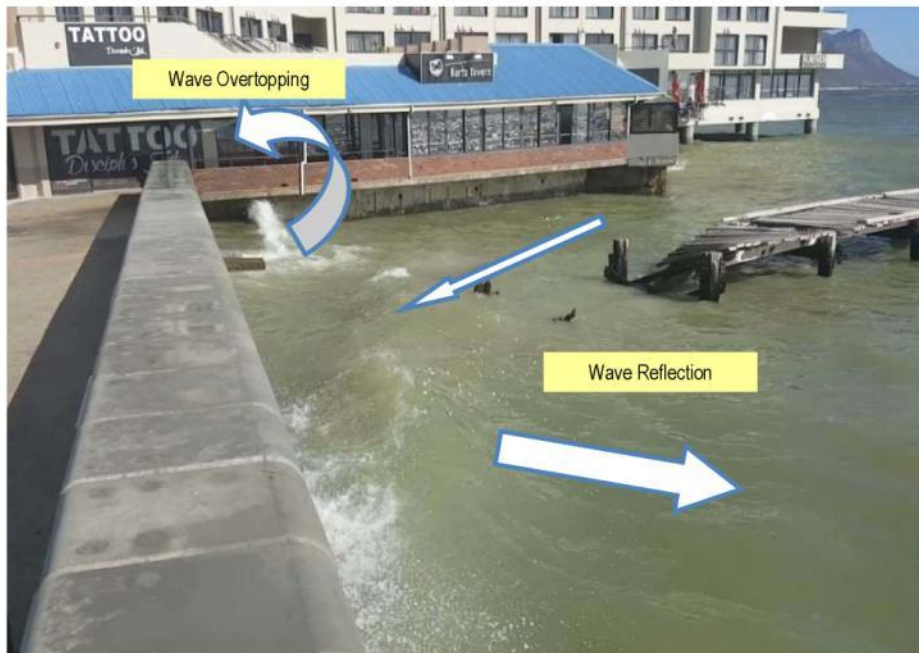
Figure 4: Wave reflection and wave overtopping at Bart's corner during MHWS - 30 January 2017
