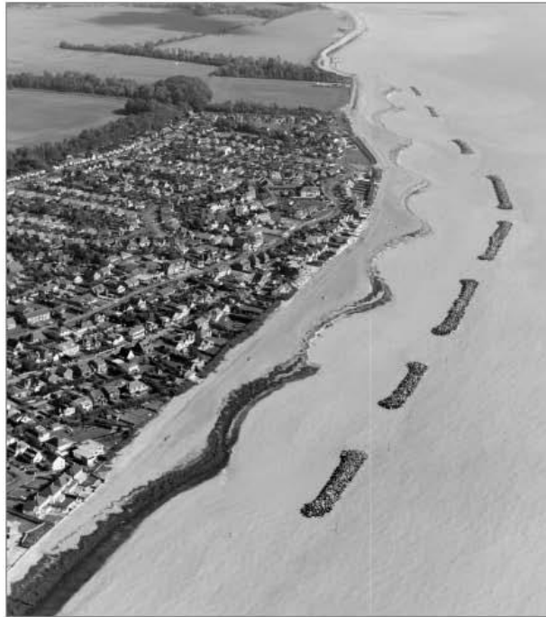
Figure 18: Example of offshore breakwaters (CIRIA, 2007)
