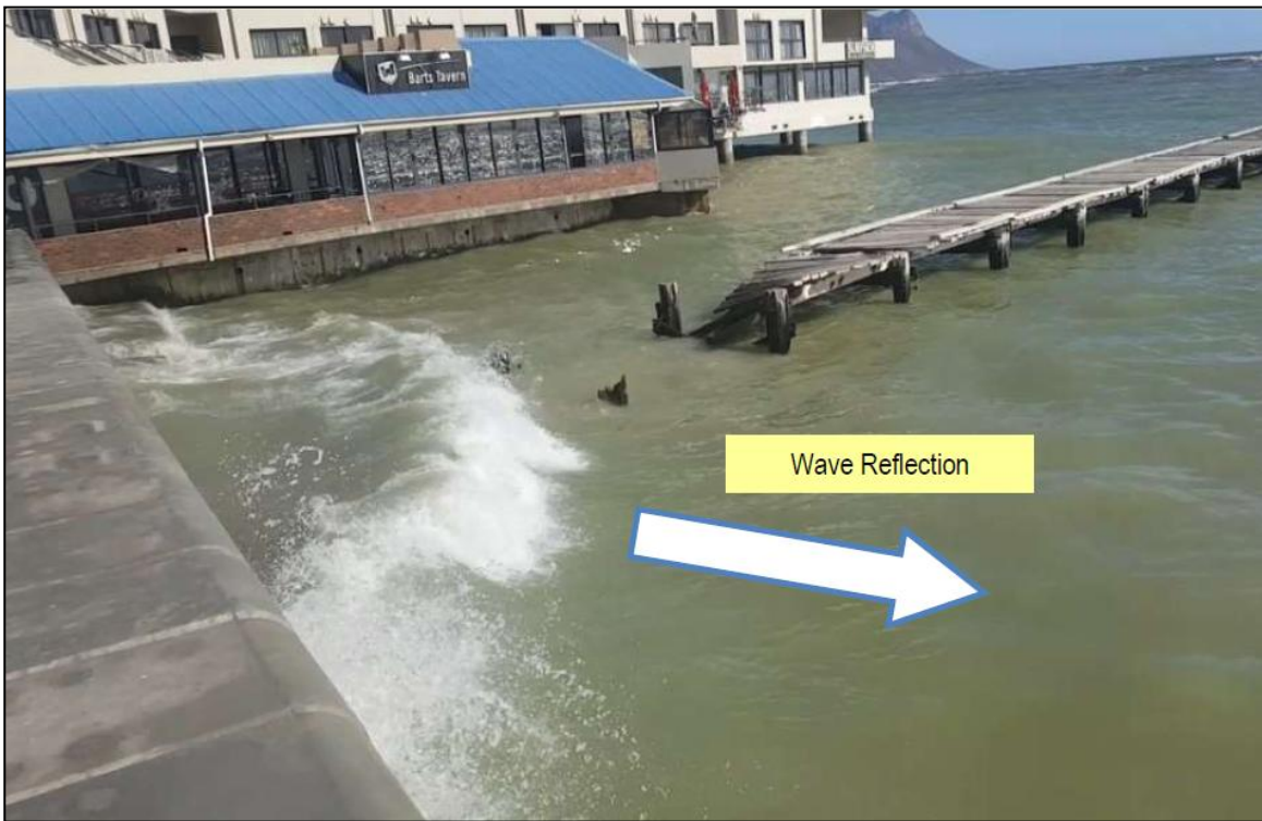
Figure 5: Wave reflection at Bart's corner during MHWS - 30 January 2017
