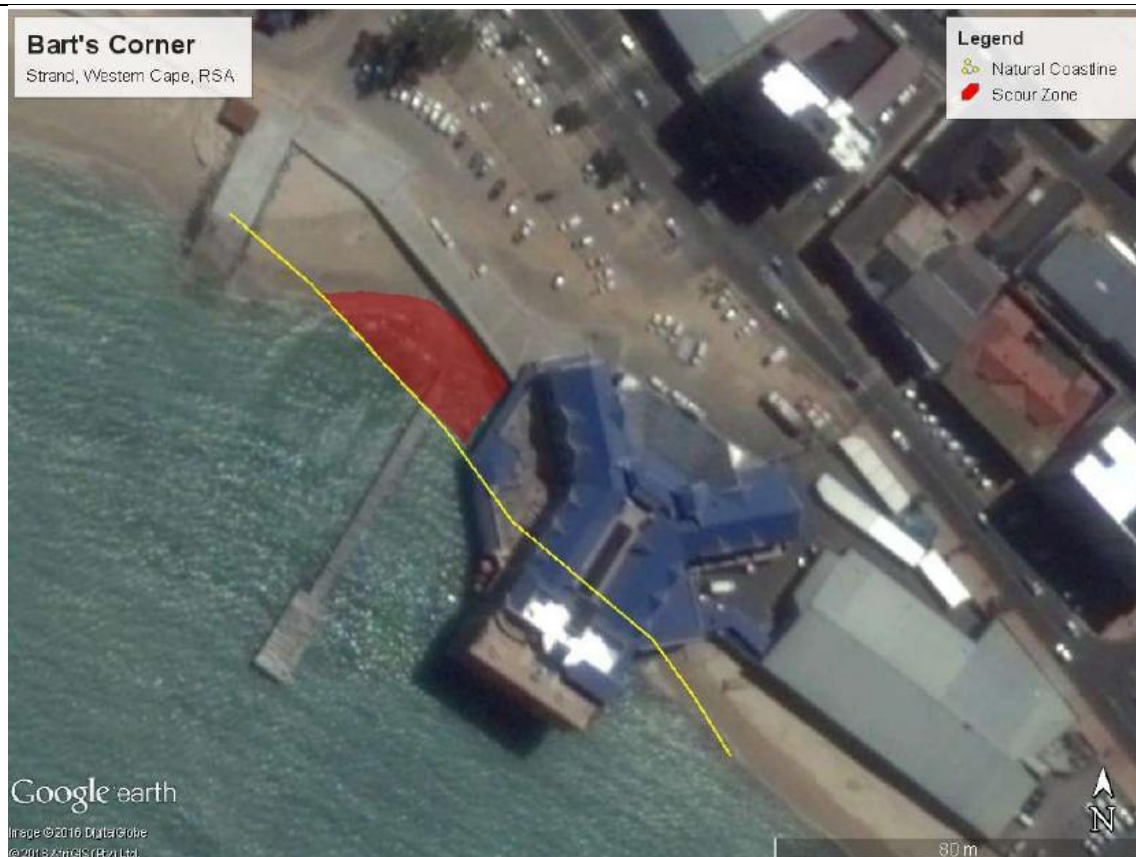
Figure 6: Aerial view of Bart's Corner. Yellow line – assumed natural coastline, red area – scour zone (Google Earth, 2017).
