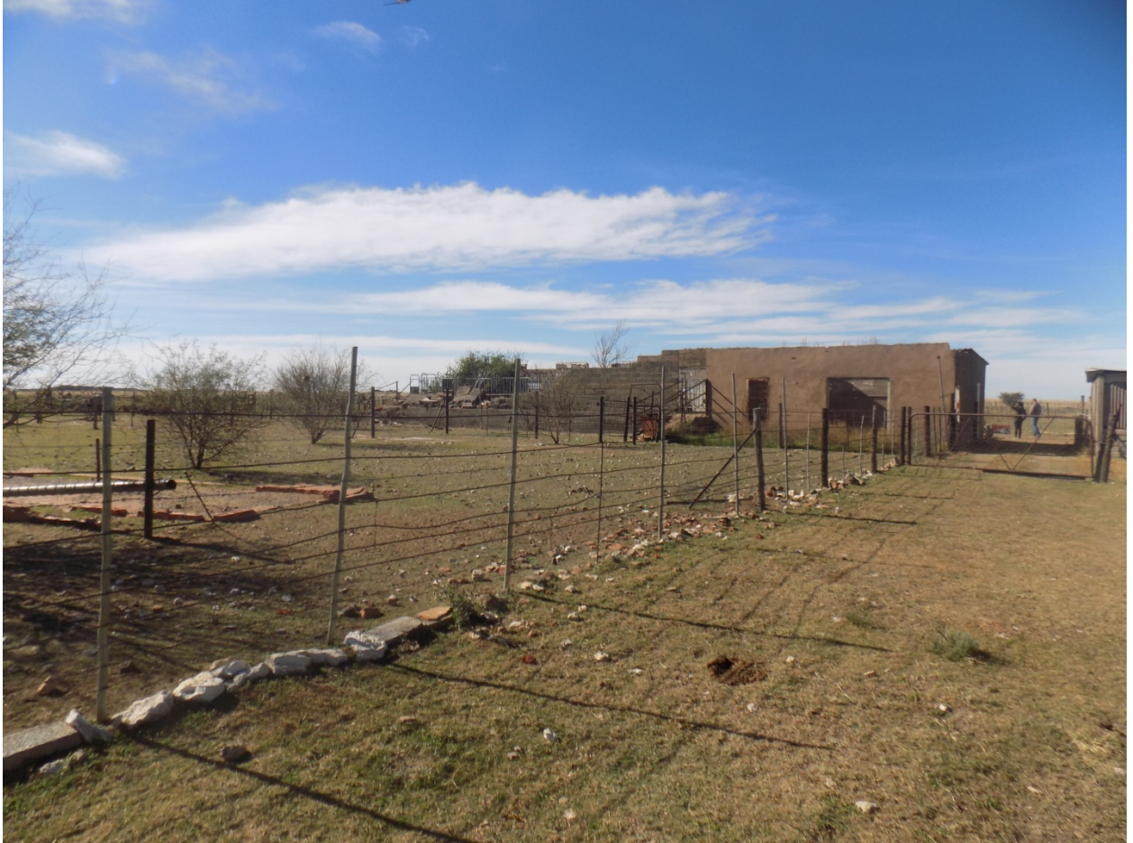
Figure 3. General view of the site, looking west.
