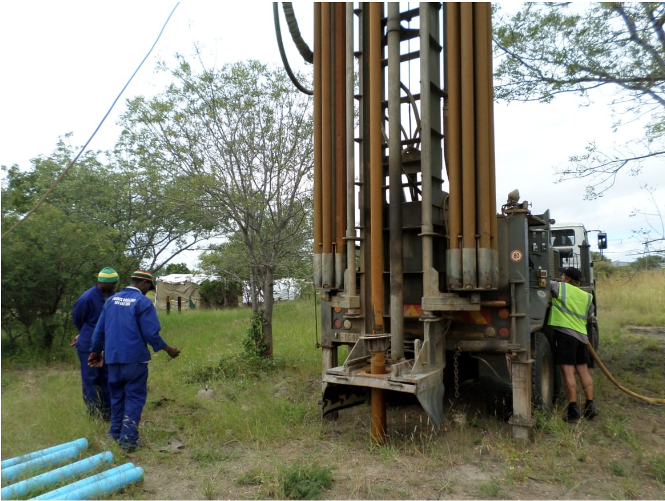
Figure 3: Example of the drilling machinery
