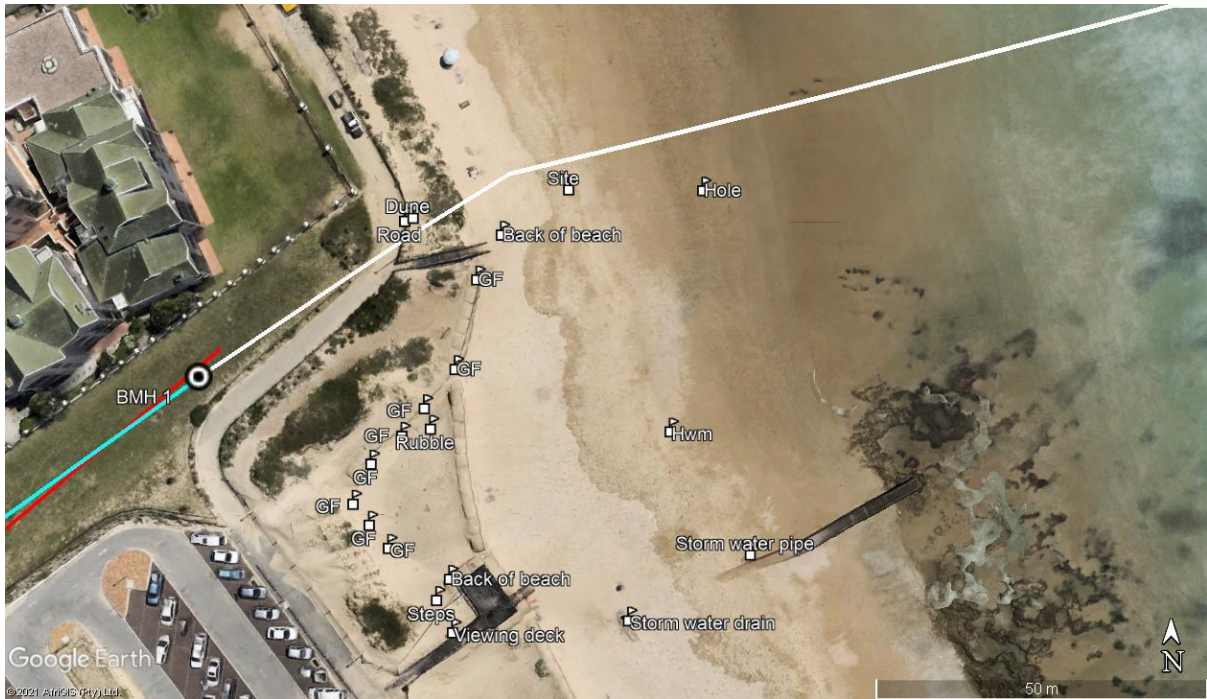
Figure 5. Image showing features identified and sample points evaluated at the cable landing point. “GF” refers to geofabric bags, a form of coastal erosion prevention.
