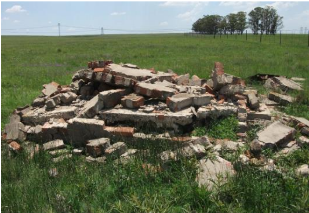
Figure 15: Pile of rubble with existing power lines in background
