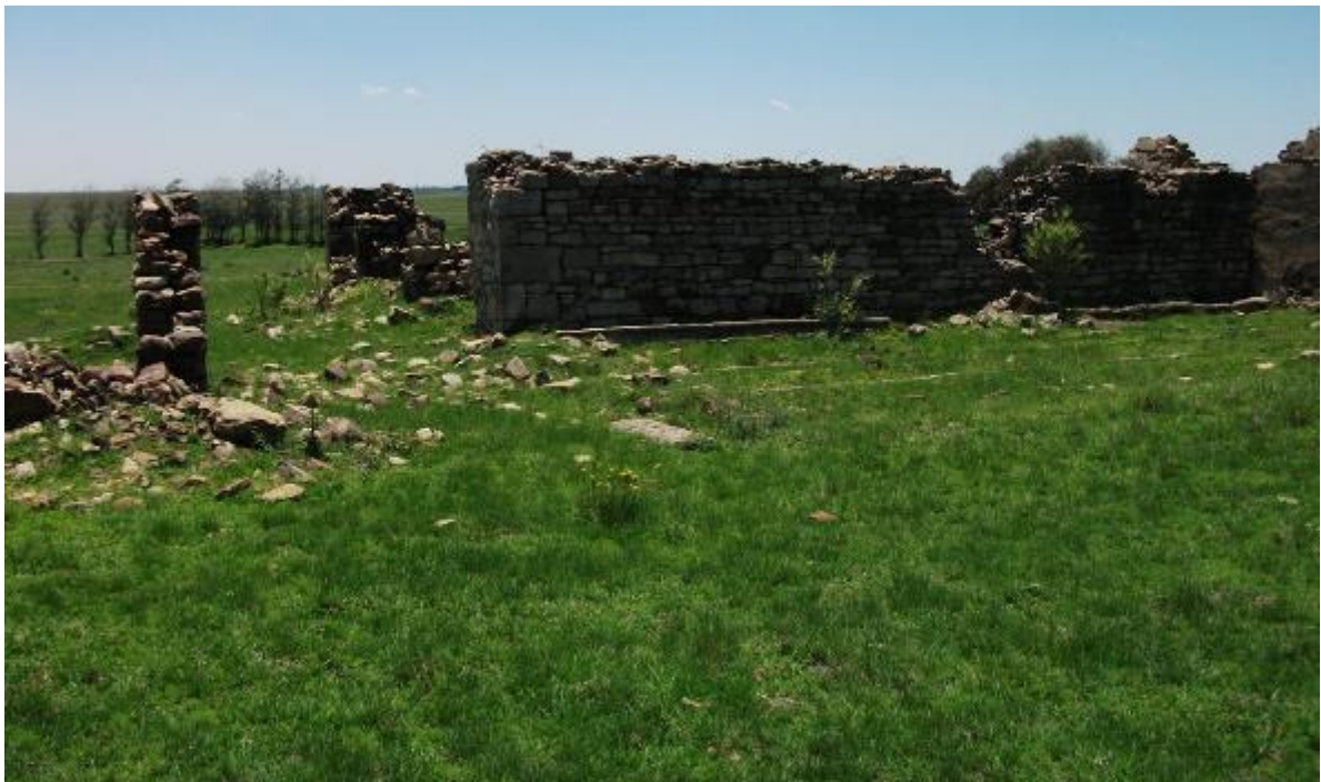
Figure 6: Remains of other structures
