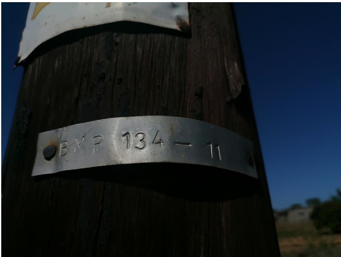
The existing pole to be connected to the proposed powerlines
