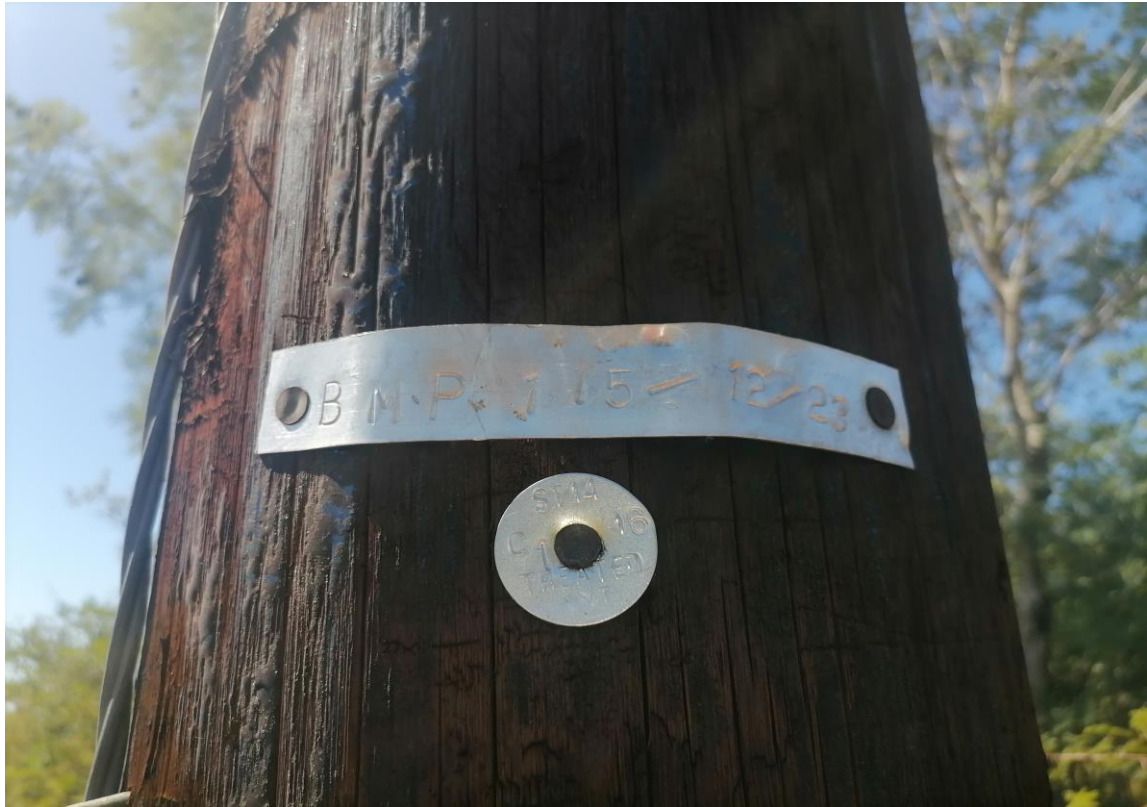
The existing pole number on site
