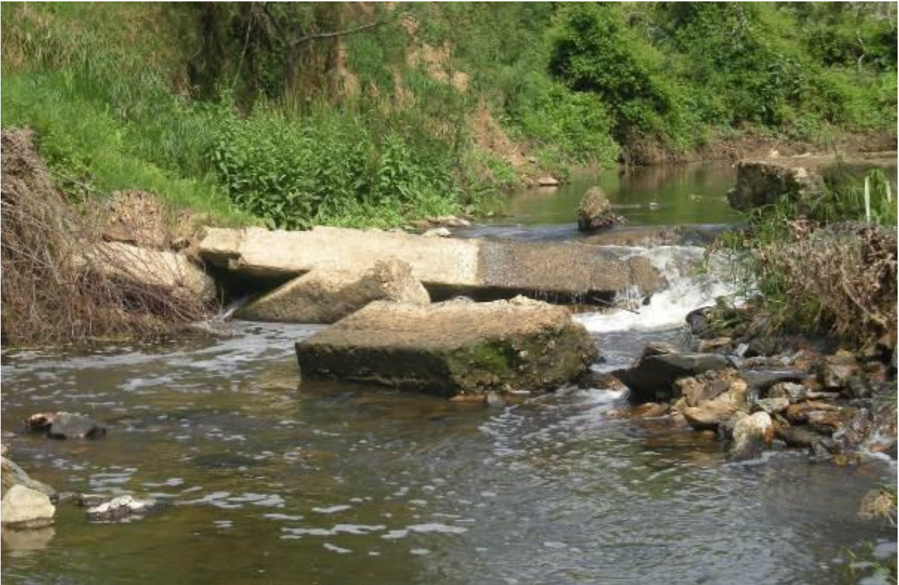
Plate 2-1: The existing weir that will be repaired.
