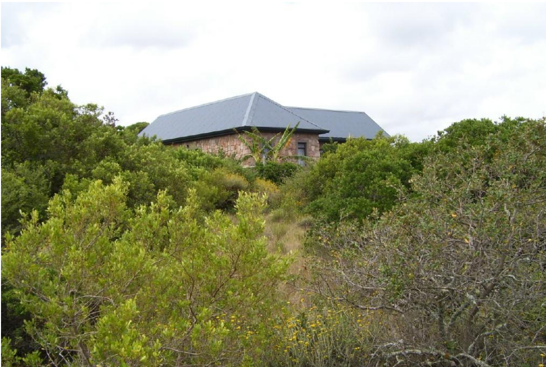
Plate 22: A green roof blends in with the vegetation
