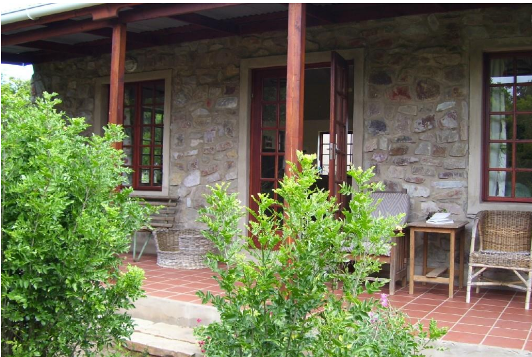
Plate 24: Wide verandas provide shade in summer, with the roof being at the correct angle to let in winter sun
