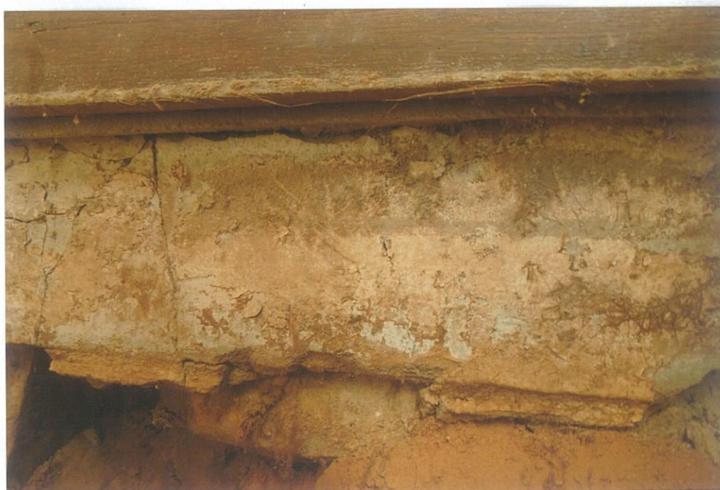
5, 6. At wall B4 even the interior wall was built-up in stone. Note the earlier floor level (c.1900) with the skirting plaster and the two yellow in situ plaster strips below, showing floor board impressions (look W) (scale 50 cm).
