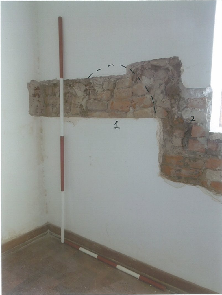
37. This southern section of Wall I4, show where the arched over opening has been filled in (1), as well as the black soot over bricks and mortar (2) (photo 38) (scales 2m, 1m) (look SW).
