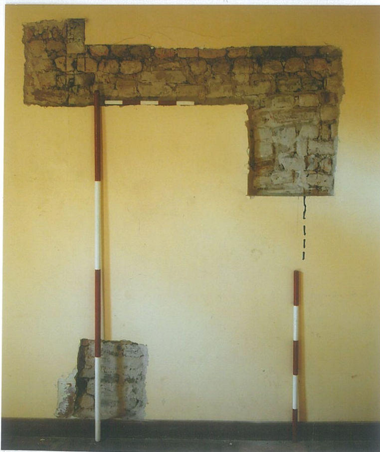
17. Close-up of the original brick versus fill-in. Its lines are traced along the filled-in brickwork (look E).
