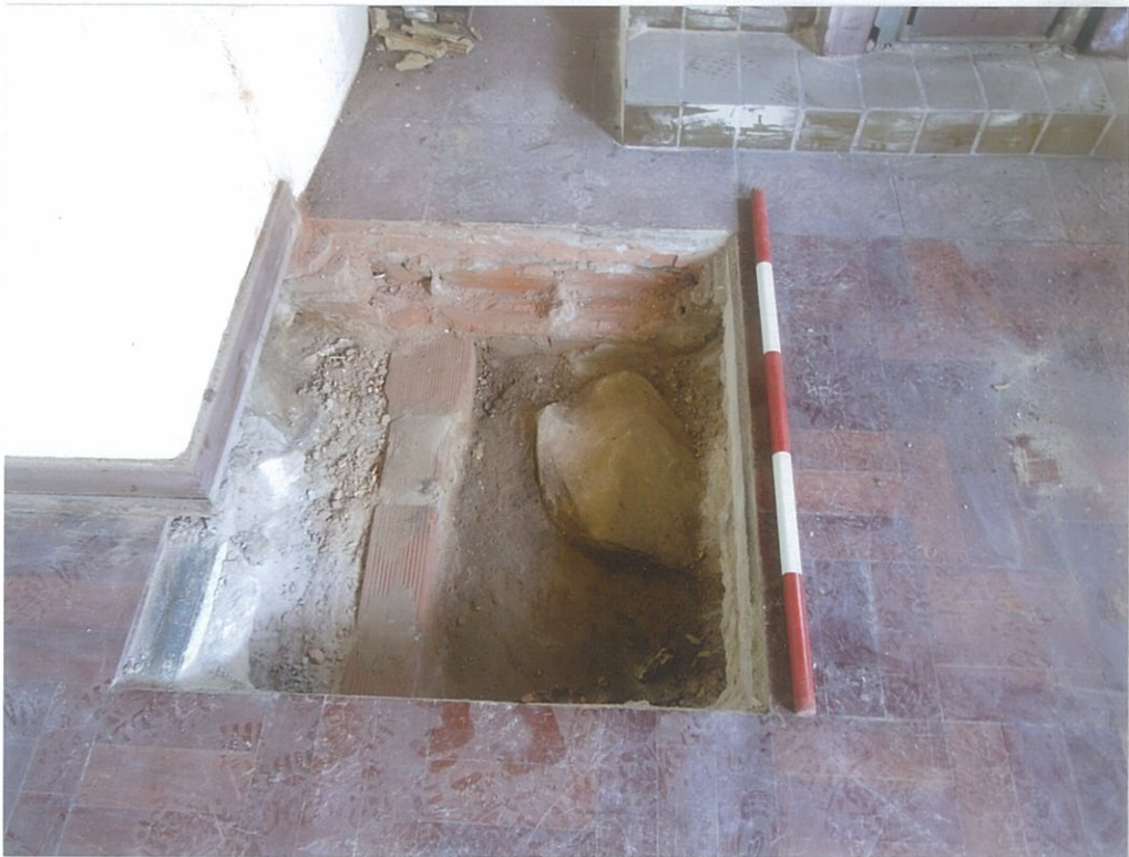
32. Next to the hearth (I3), another section also exposed the 1940 bricks (1) and a large stone (2), probably part of an earlier foundation (scale 1m) (look S).
