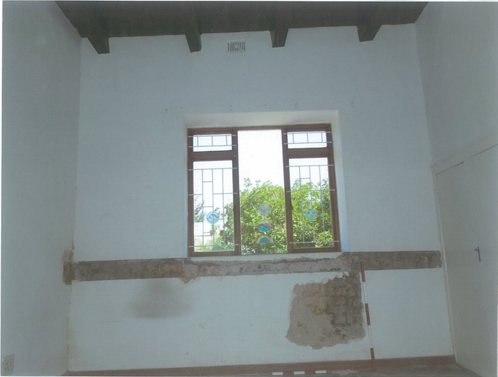
27, 28. View in Room G ( Agterkamer ) of wall G4 and the plaster stripped. Note in the close-up the older 18 th c brick (1) and the filled-in brick and yellowish mortar on the left (2) (look W) (scales 1m, 50 cm).
