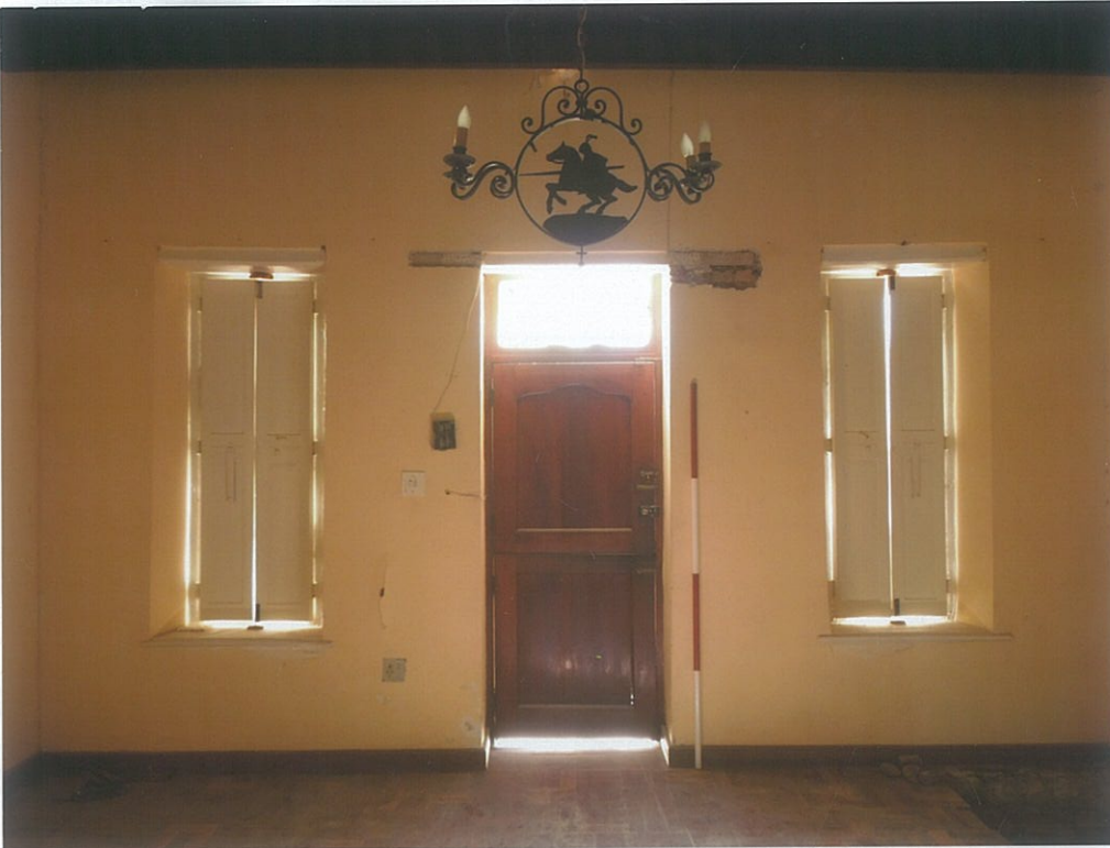
10. View in Room C, showing the front entrance (C1). Note the exposed lintel above the bright fanlight (look N).
