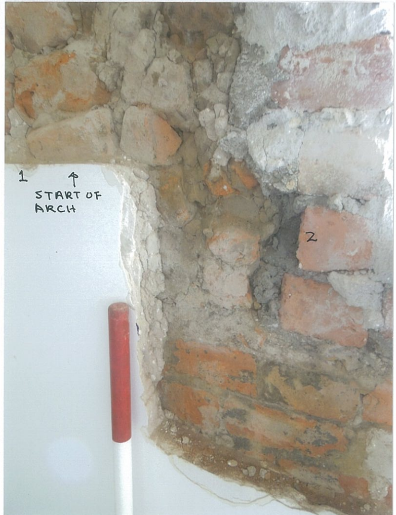
37. This southern section of Wall I4, show where the arched over opening has been filled in (1), as well as the black soot over bricks and mortar (2) (photo 38) (scales 2m, 1m) (look SW).
