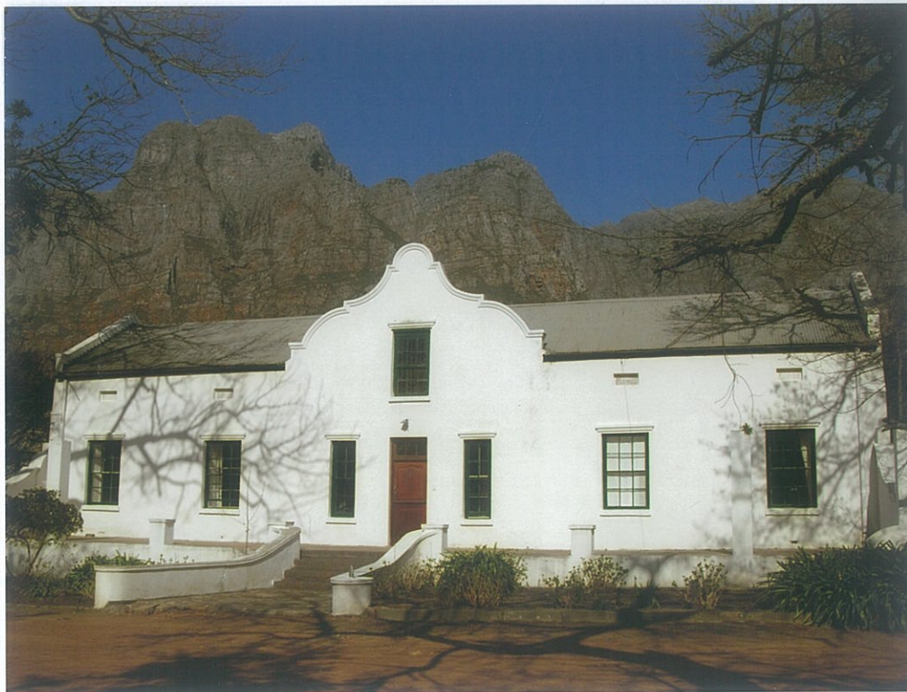
48. View of the Homestead, where the broad stoep and entrance staircase lend some status to the plain facade (look S).
