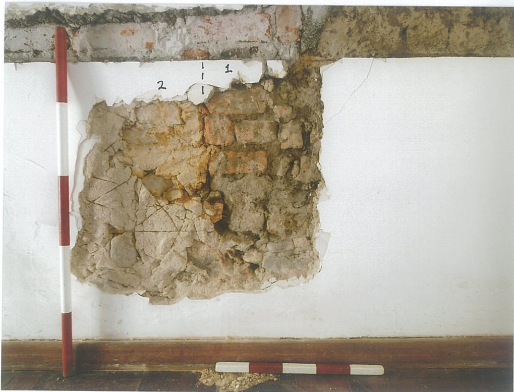
27, 28. View in Room G ( Agterkamer ) of wall G4 and the plaster stripped. Note in the close-up the older 18 th c brick (1) and the filled-in brick and yellowish mortar on the left (2) (look W) (scales 1m, 50 cm).
