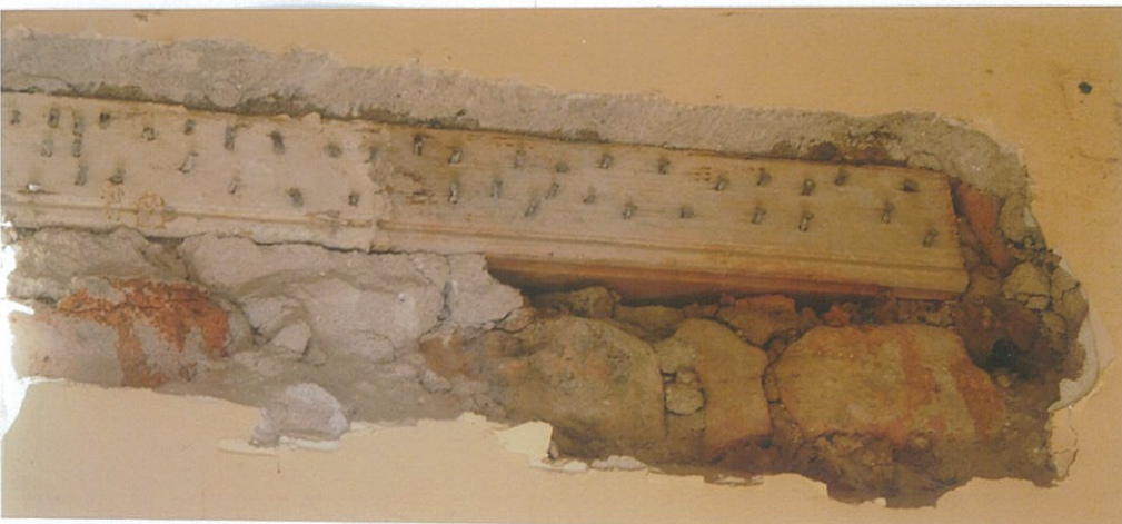
12. The right portion of painted lintel versus unpainted (look N).
