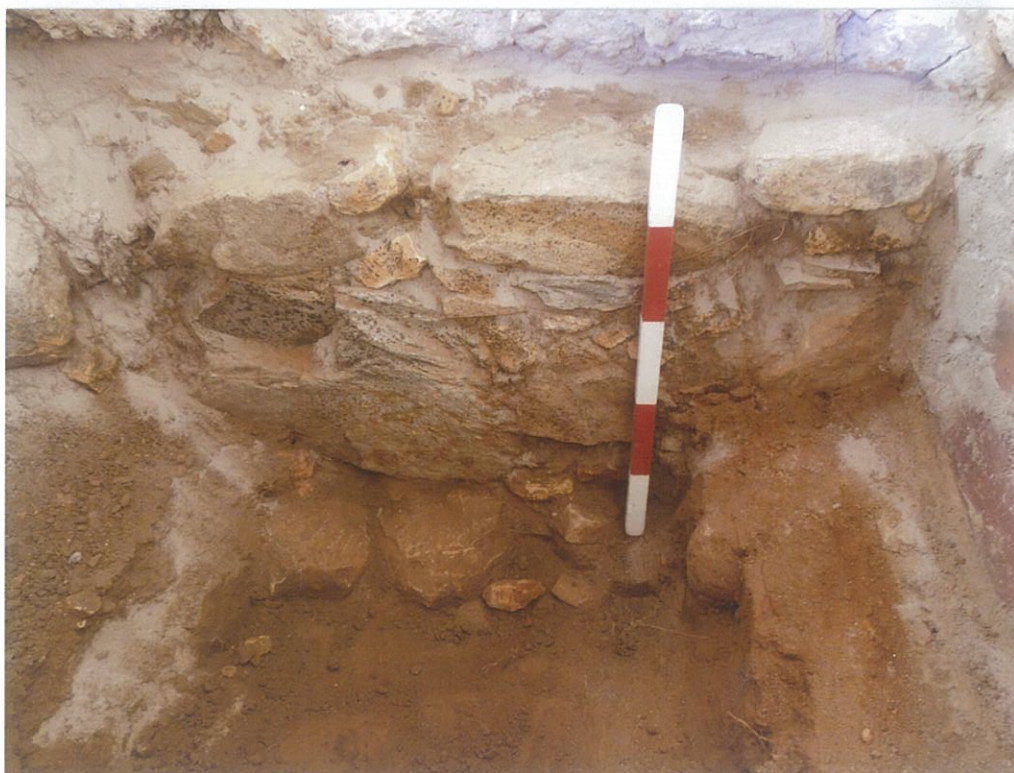
9. Same view, exposing the lower plinth of stones as a rough base for the upper granite foundation (look N) (scale 50 cm).
