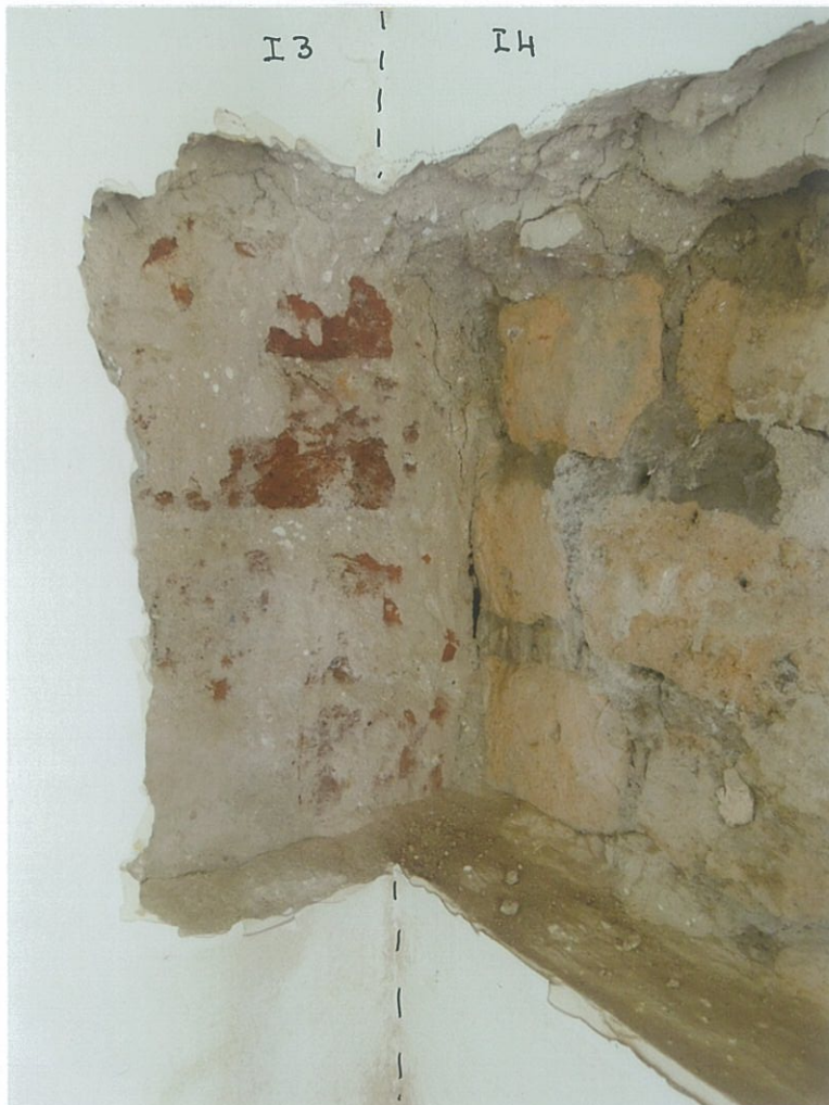
36. Corner section, where the hearth wall I3 shows modern brickwork on the left (look S).
