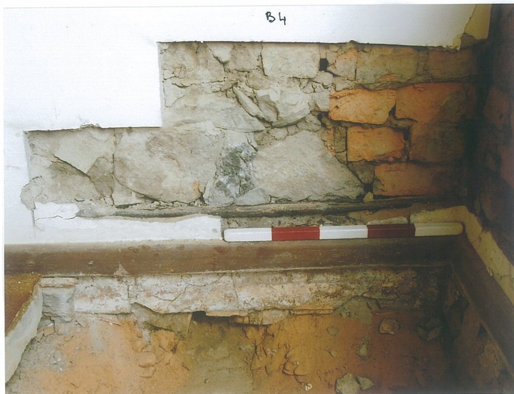
5, 6. At wall B4 even the interior wall was built-up in stone. Note the earlier floor level (c.1900) with the skirting plaster and the two yellow in situ plaster strips below, showing floor board impressions (look W) (scale 50 cm).
