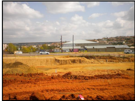
Figure 6: View from the site facing north-west
