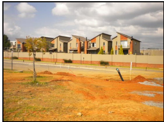
Figure 10: General site conditions
