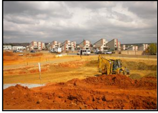
Figure 4: View from the site facing West
