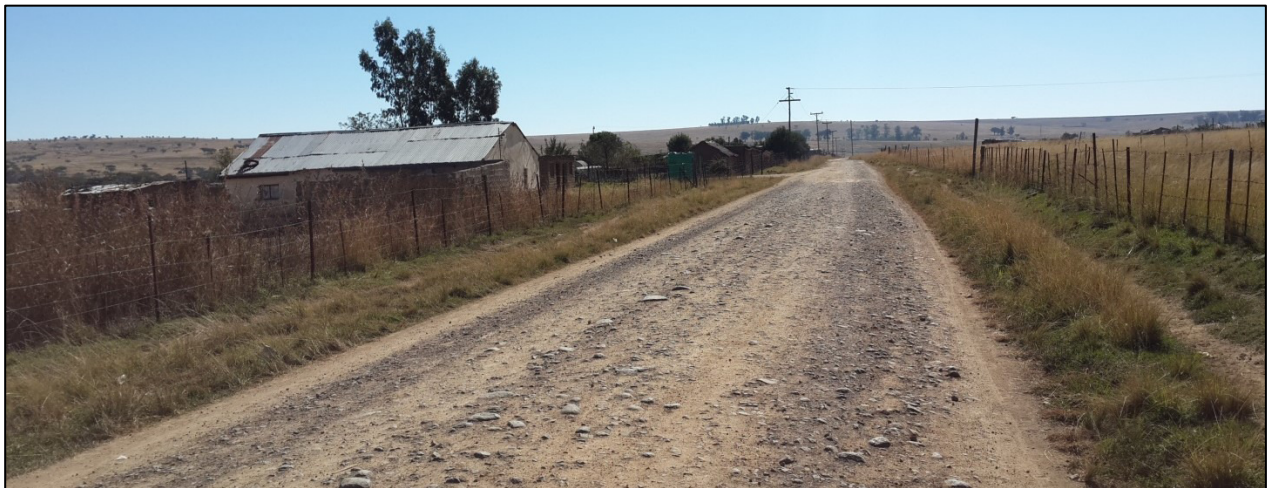
Plate 4: An example of the road network adjacent to which pipelines will be laid
