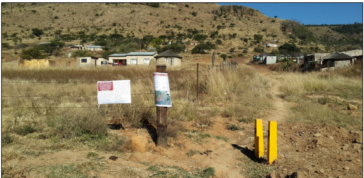
Plate 5: The footprint of an existing bulk pipeline, adjacent to which the new pipeline will be established, limiting the impact on the receiving environment
