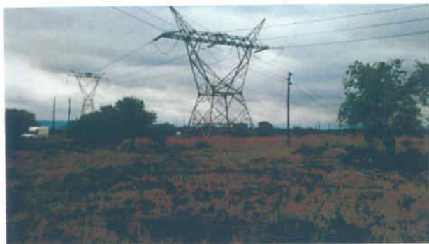
Road South of Bighorn Substation
