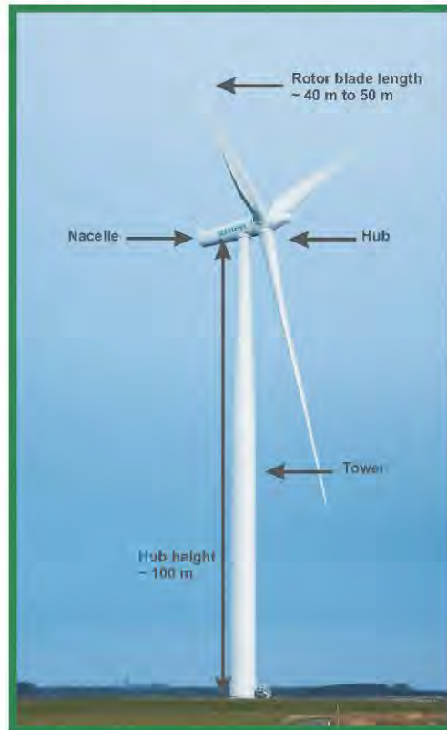
Figure 1: Siemens 2.3 MW wind turbine, which is indicative of the type of wind turbine envisaged for this project.
