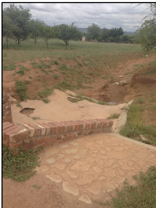
Photo 4: Stormwater drain along D620 route
