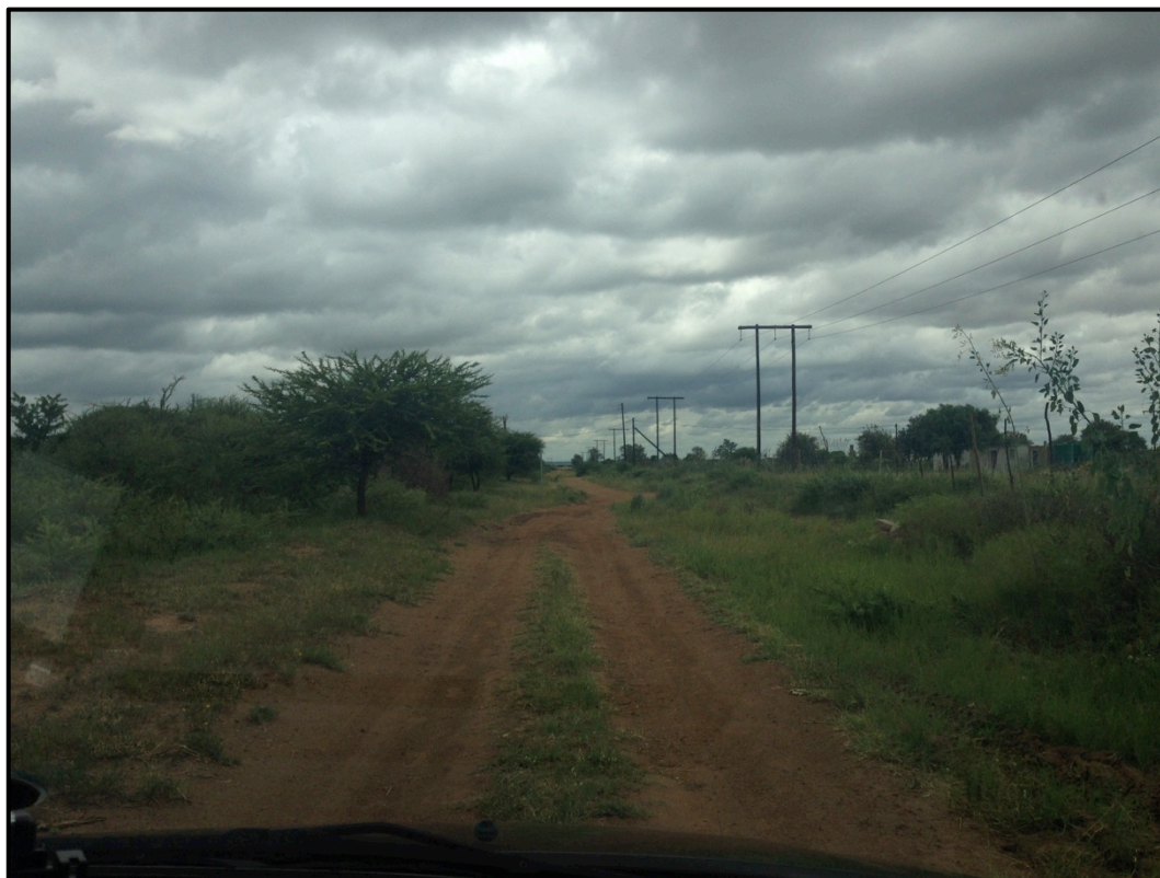
Photo 3: Gravel road (D620) at about 7km looking north
