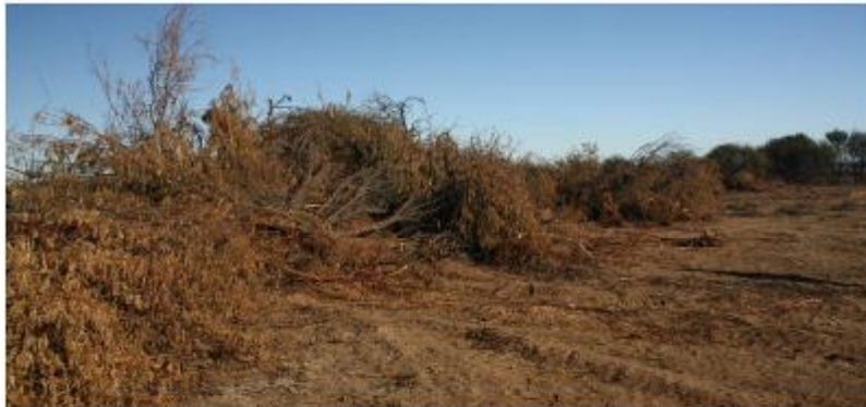
Figure 8: Large amount of vegetation cleared from the site.
