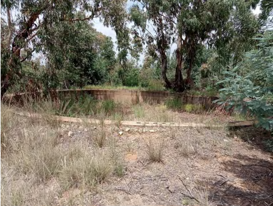
FIGURE 16: VIEW OF RESERVOIR AT SITE 3.
