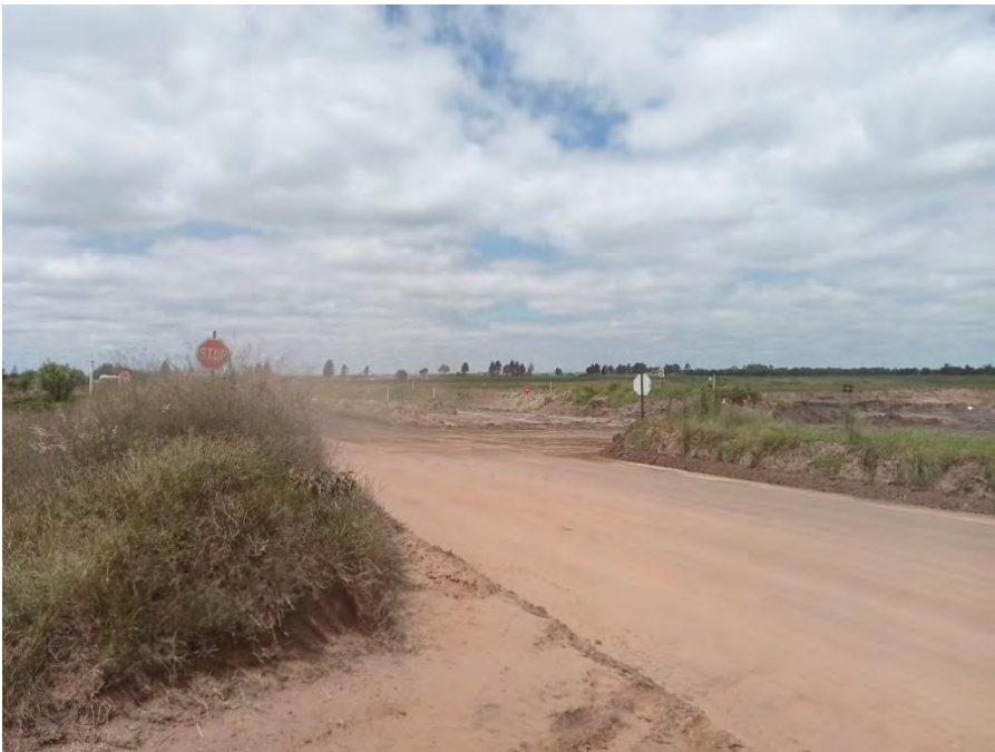
FIGURE 6: VIEW OF A DIRT ROAD USED BY MINING TRUCKS IN THE SURVEYED AREA.
