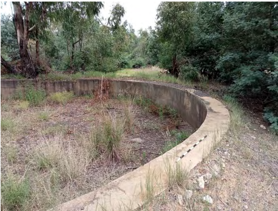
FIGURE 17: CLOSE UP VIEW OF THE RESERVOIR.
