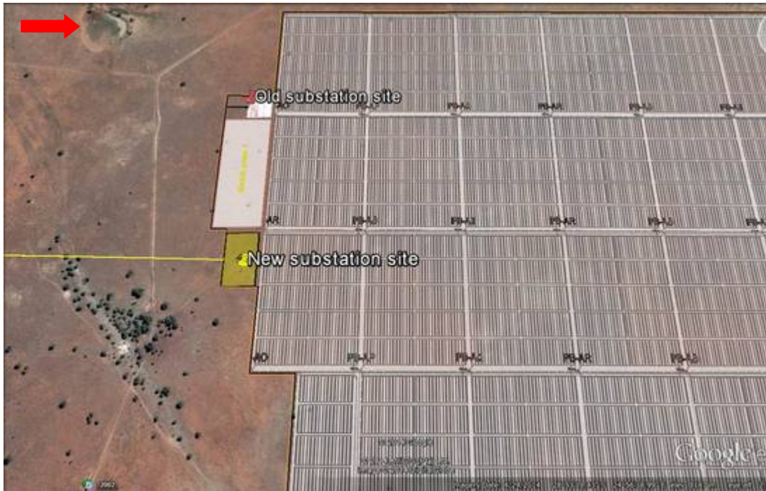
Figure 2: The on-site substation moved 500m south to its current position to avoid one of the power line alternatives (yellow line) from crossing a pan located north-west of the substation (indicated by the red arrow).
