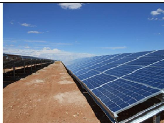
Figure 2.4: Picture of a PV Panel
