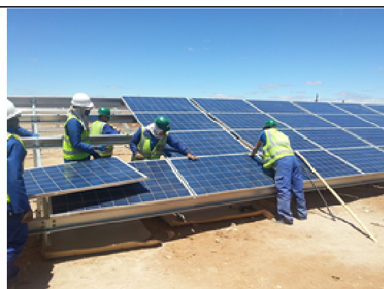
Figure 2.5: Picture of the installation of a typical PV array
