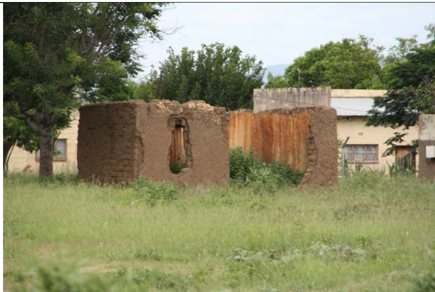
Old structure build with mud walls
