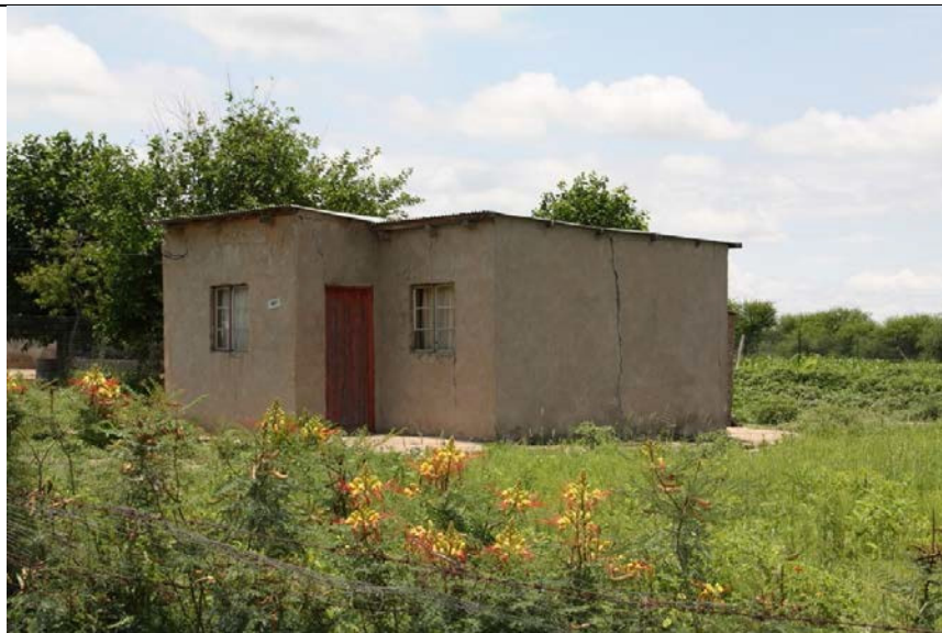
House with very prominent vertical crack
