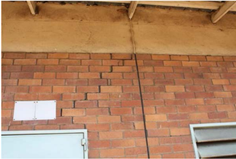
Figure 12: Example of blast induced damage.
