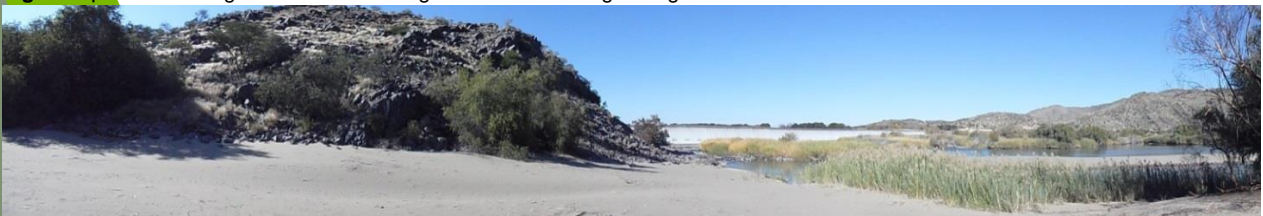
Figure 5 | Photo of the proposed position of the powerhouse on the Orange River.
