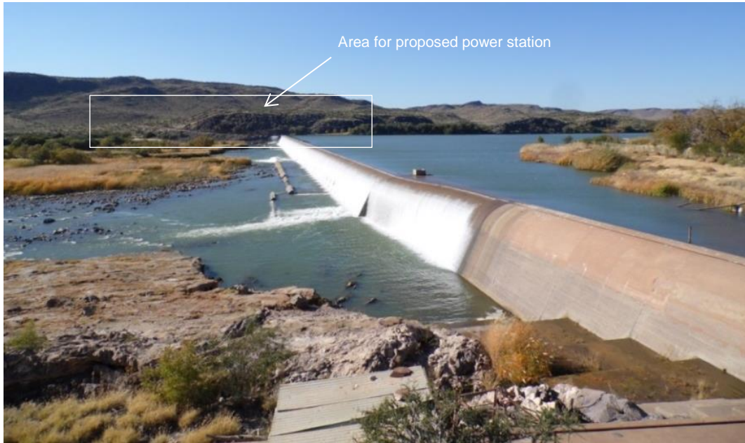
Figure 7 | Boegoeberg weir, taken from the southern bank. The power station would be situated on the northern bank.
