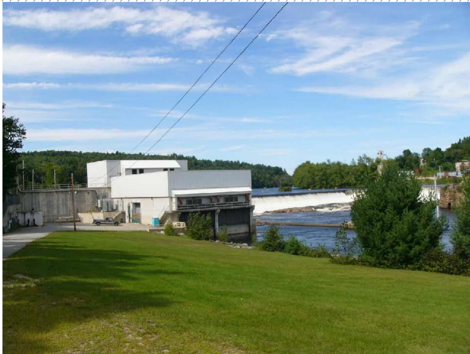
Figure 14 | Example of a power house. (Source: http://www.lowimpacthydro.org/ Accessed: 28 June 2013).
