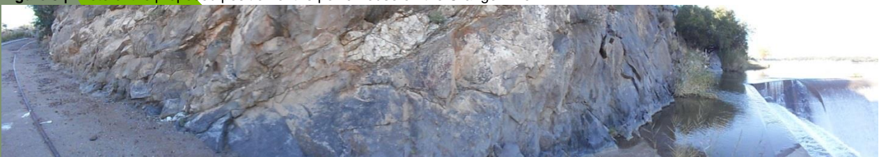
Figure 6 | Photo where the proposed channel/pipeline will be excavated from the rock face.
