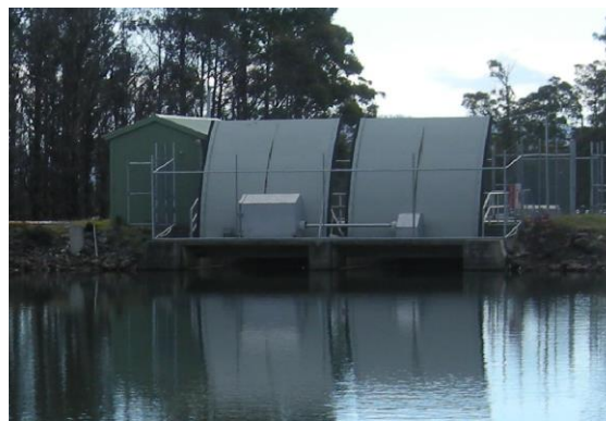
Figure 8 | Example of a similar intake structure with trash racks and cleaner. The proposed intake would not have the gate shed.
