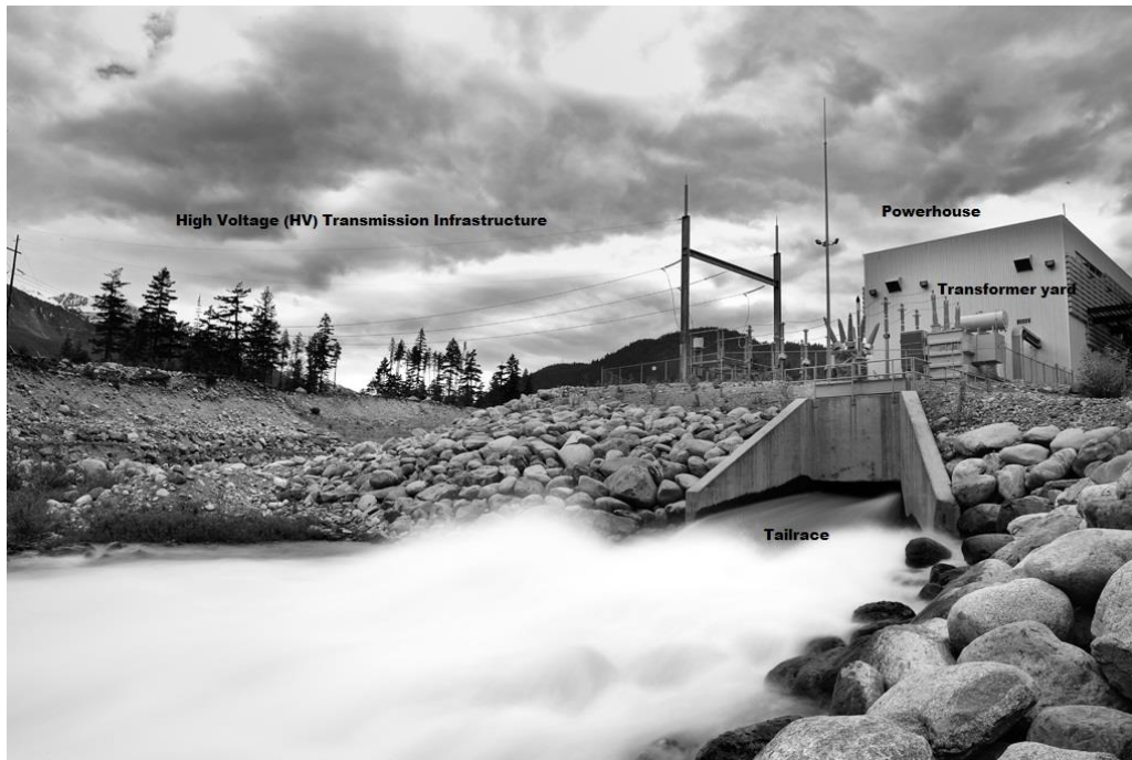
Figure 5 | Example of a powerhouse, transformer yard, transmission and tailrace infrastructure. source: http://www.photosensitive.com (Accessed: 28 June 2013)].
