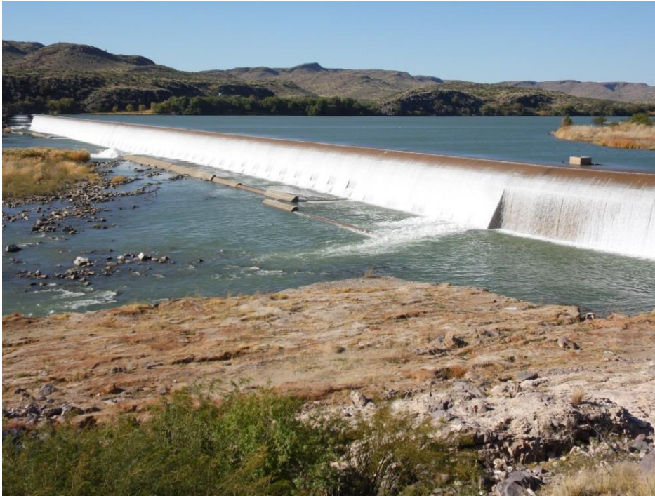
Figure 32. Boegoeberg Dam from the south bank
