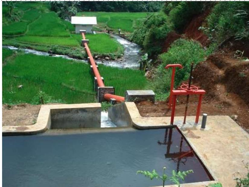
**Figure 11** | Example of a small head pond. (Source: energypedia.info (Accessed: 28 June 2013)).
