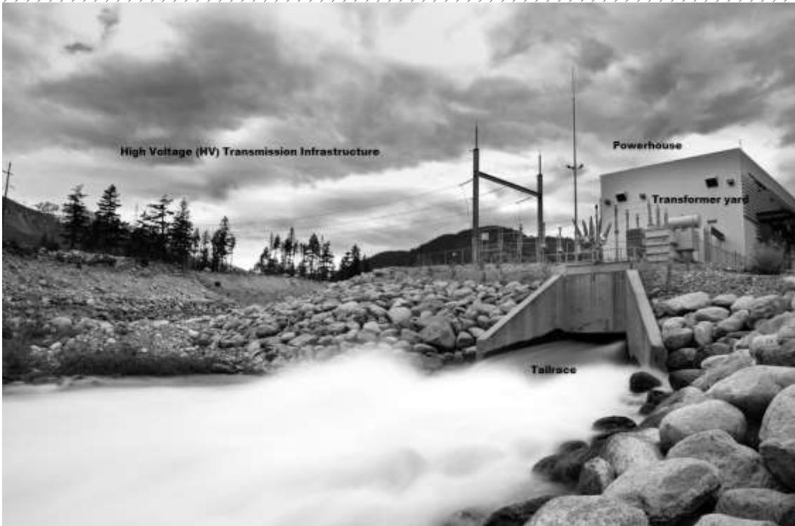
**Figure 17** | Example of a powerhouse and associated infrastructure. (source: <http://www.photosensitive.com> (Accessed: 28 June 2013)).
