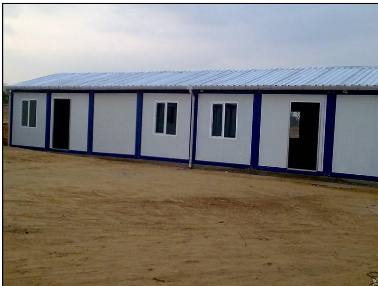
Figure: Typical office and accommodation block
