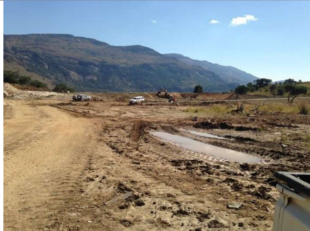
2-5a) New Pollution Control dam at the Valley Boxcut
