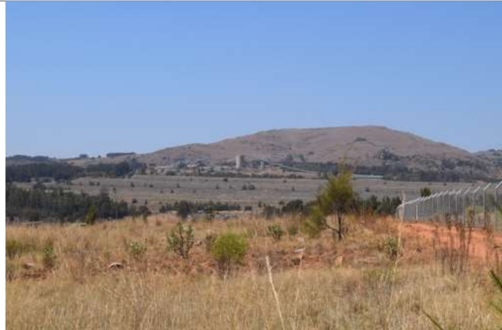
2-5c) Existing Tailings Storage Facility at BS4 to be reworked
