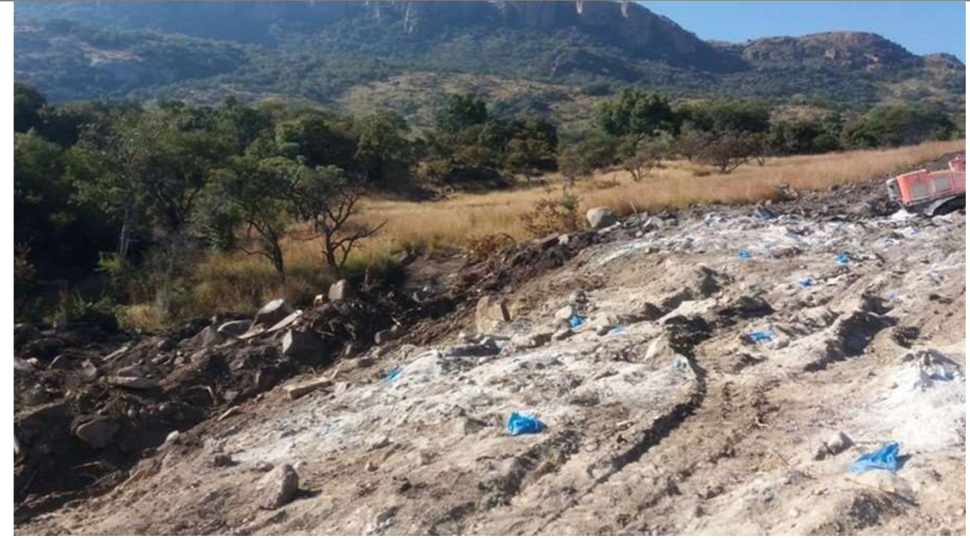
2-11d) Road Clearance through a Seep Wetland at BS4
