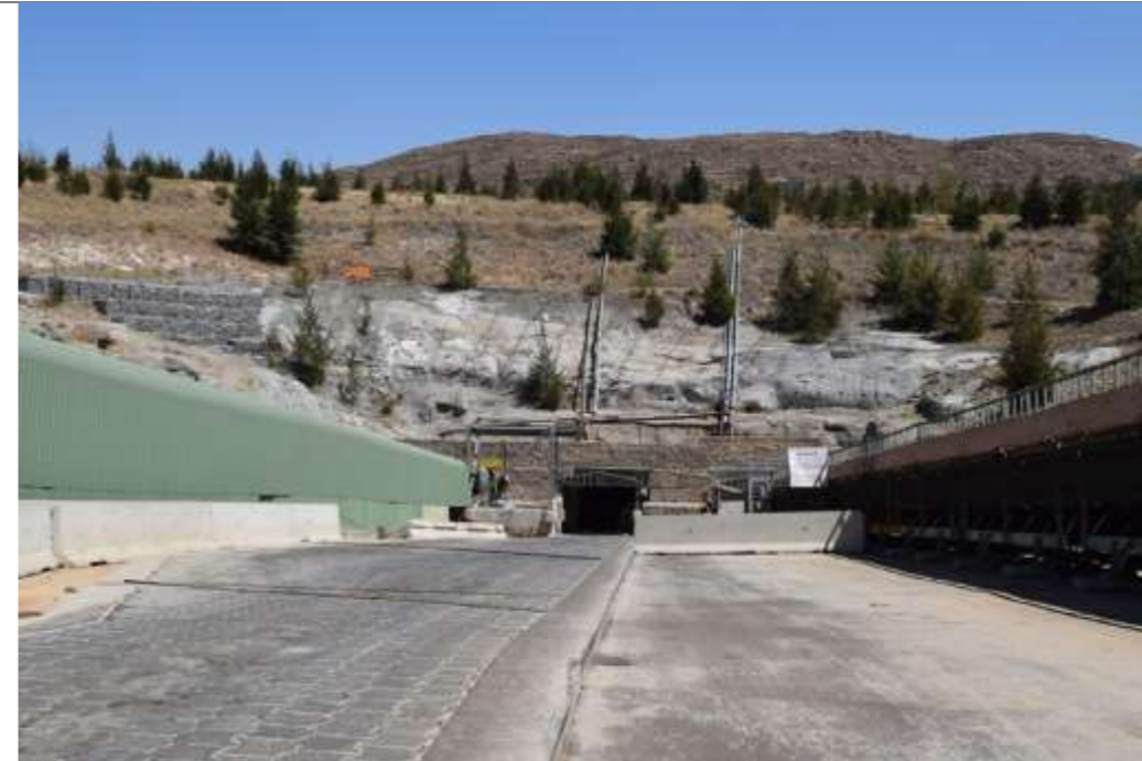
2-5d) Underground Workings at BS4 to be Backfilled with Tailings
