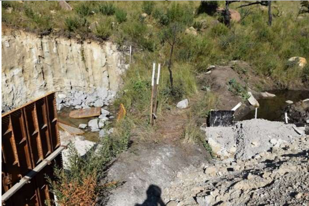
2-11g) Construction within the Waterfall River Crossing (upstream)
