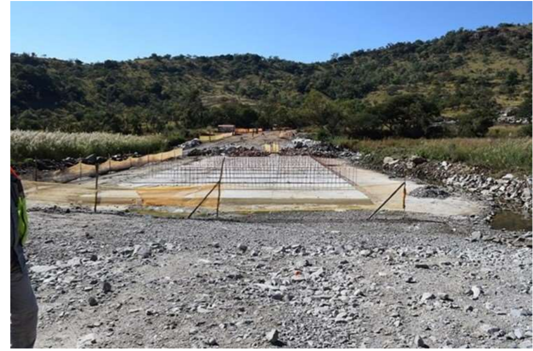
2-11f) Construction of the Groot Dwars River Crossing
