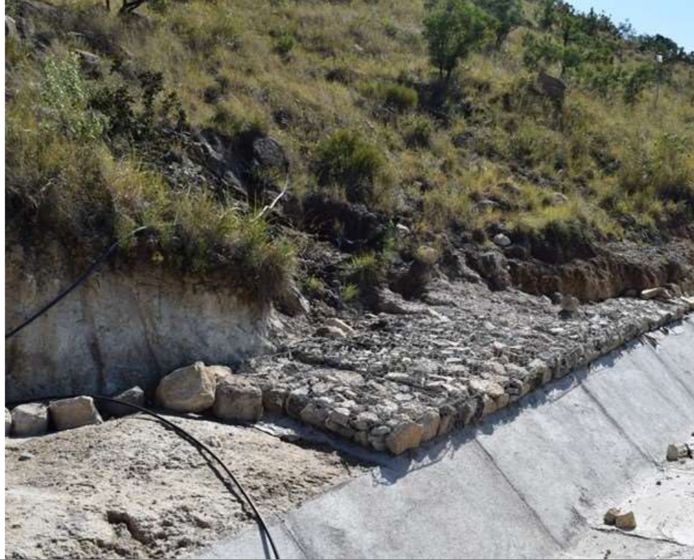
2-3e) Upstream Stream Diversion and Cut-off Trench
