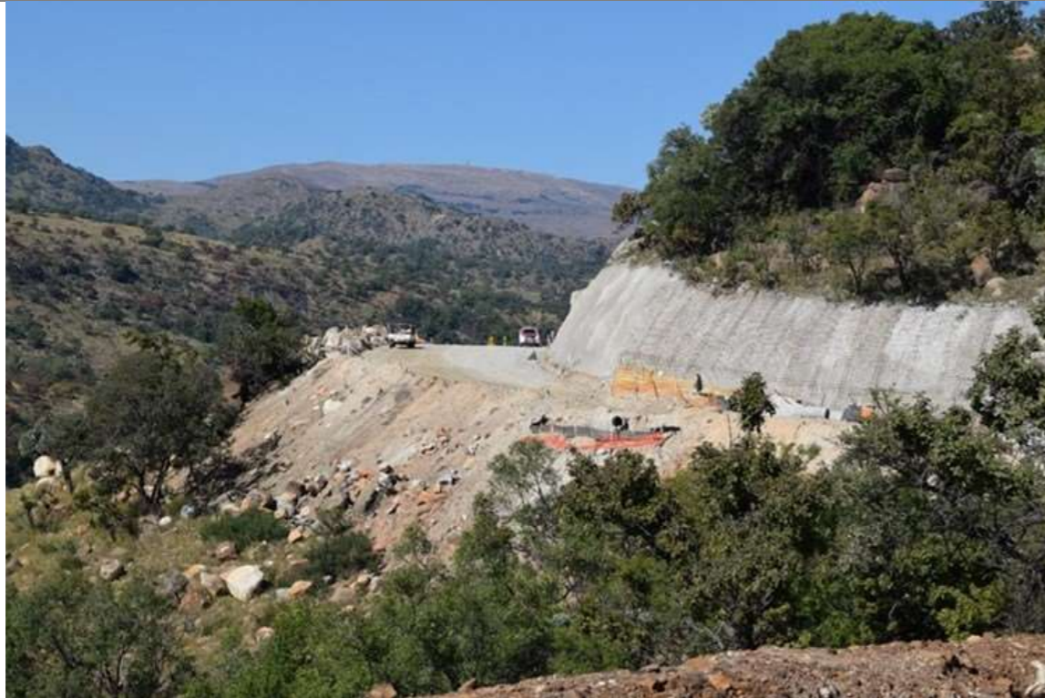
2-11c) Stabilisation of Steeper Section between BN and BS1/2
