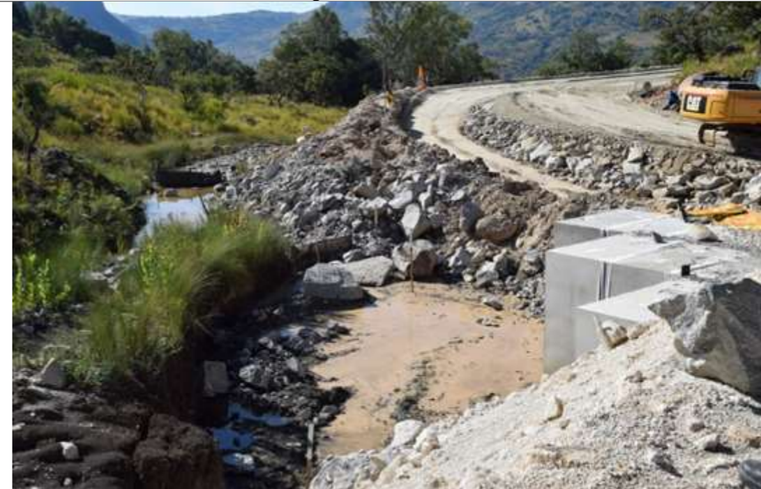
2-11h) Construction within the Waterfall River Crossing (downstream)
