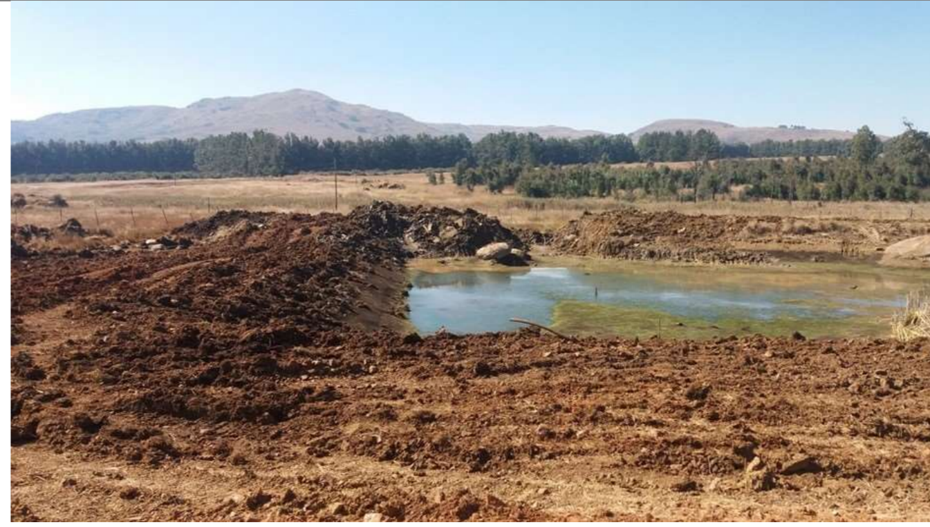
2-5b) Upgrade of Mine Pollution Control Dam 1 (MCC1) at BS4
