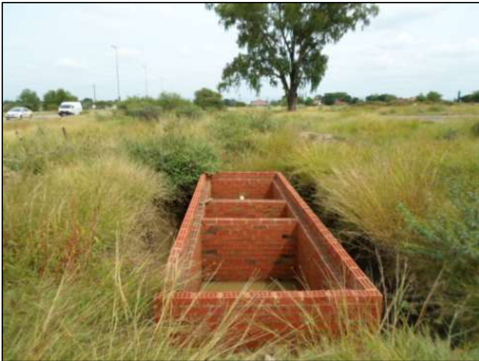
Figure 24. Existing pipeline running alongside the proposed water pipeline.
