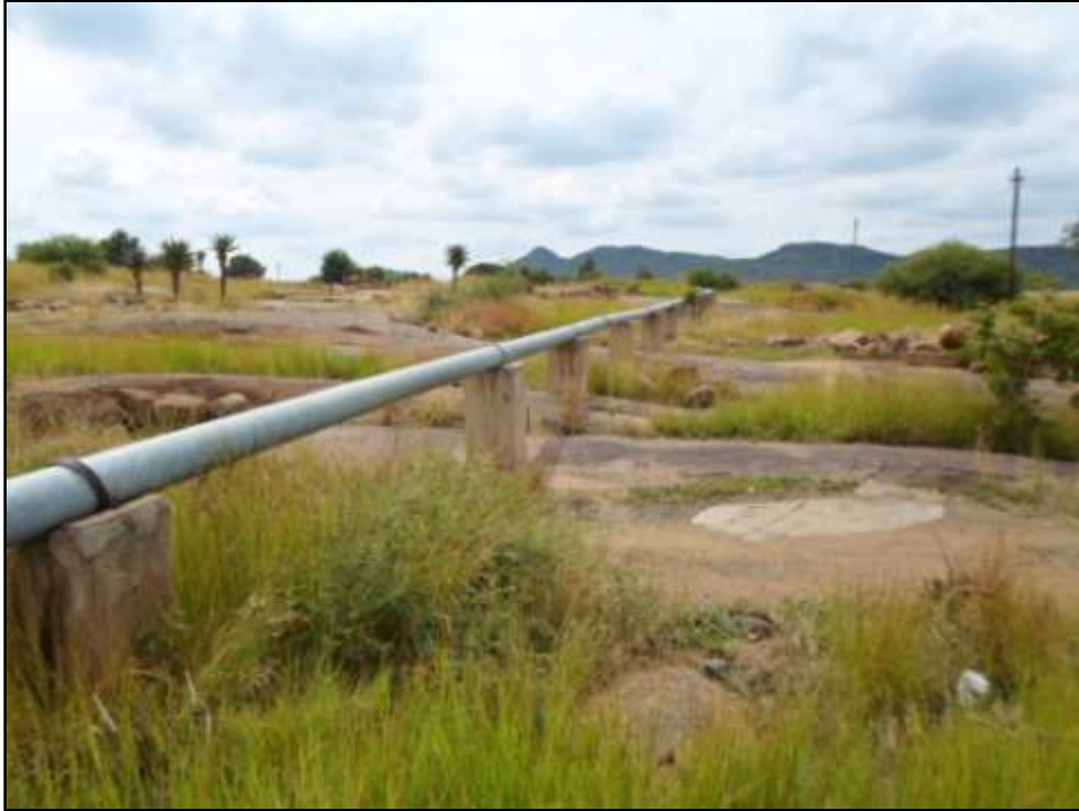
Figure 23. Existing pipeline running alongside the proposed water pipeline.
