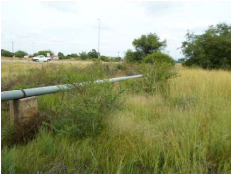
Figure 22. Existing pipeline running alongside the proposed water pipeline.
