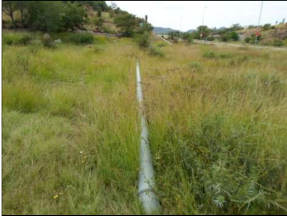
Figure 21. Existing pipeline running alongside the proposed water pipeline.
