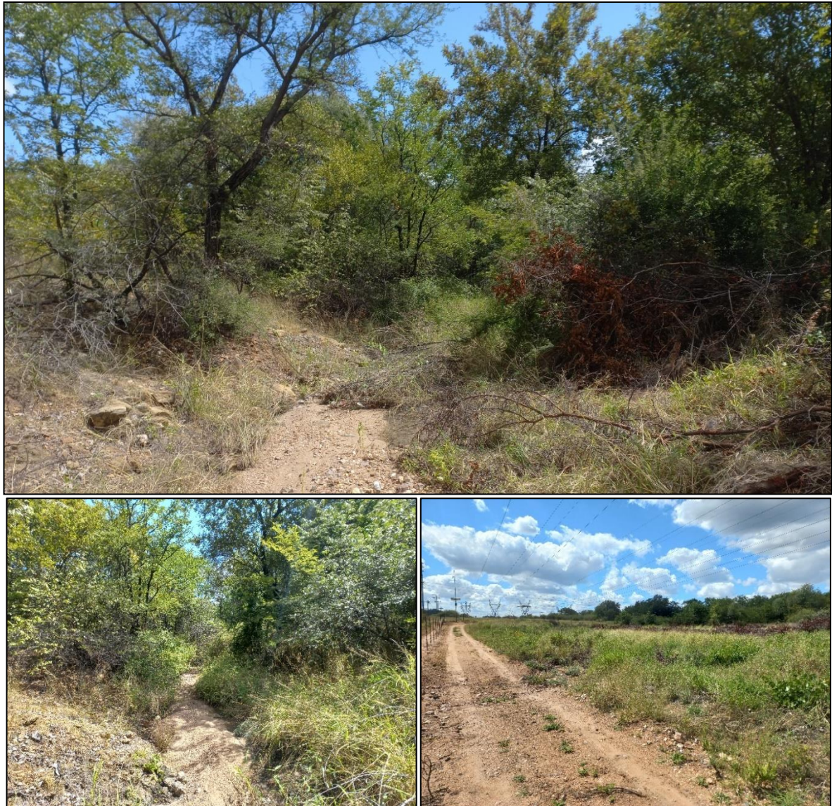
Figure 7.4.10.1(d): Bottom right shows vegetation clearing under the powerline across the riparian habitat.
