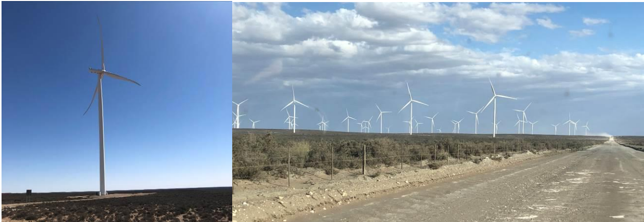
Figure 2-4: Example of an operational wind farm.
