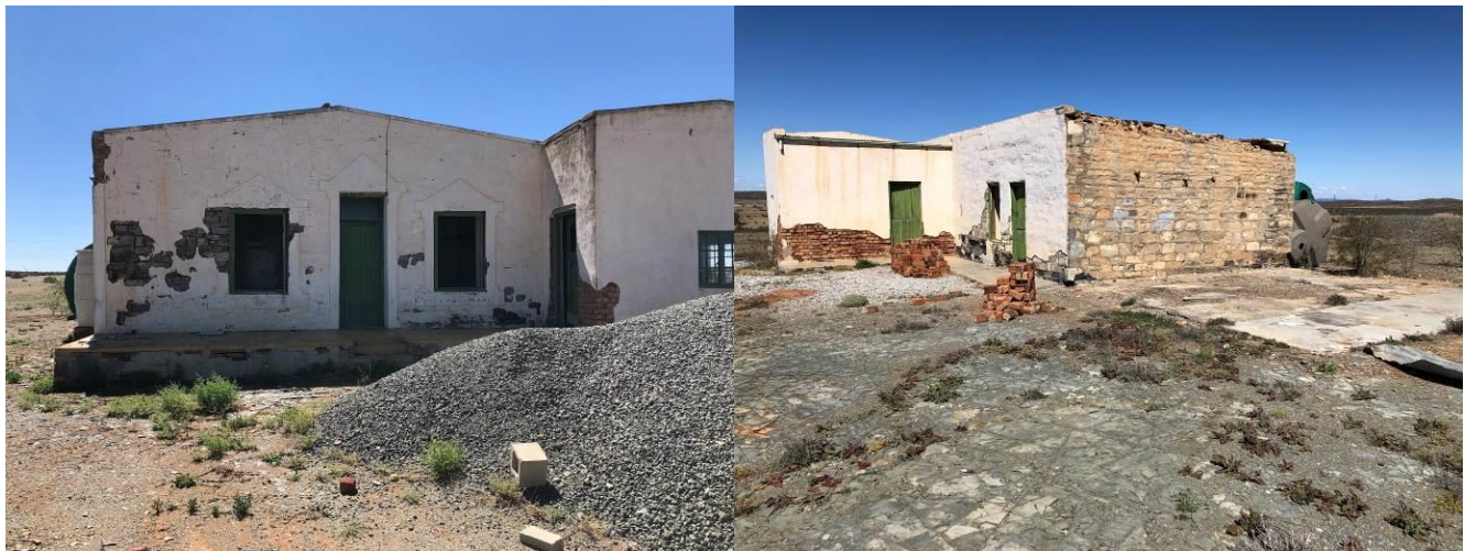
Figure 5-7: Abandoned farmstead on the study area.
