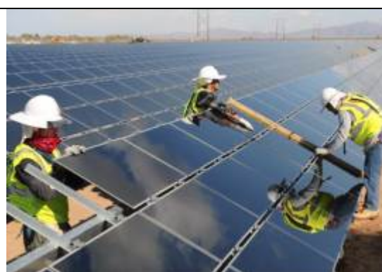
Figure 2.4: Picture of the installation of a typical PV array
