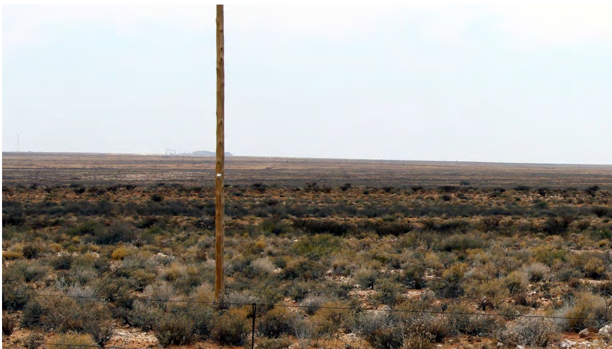
Figure 7-15 View from photo site SCA014 eastwards. The tower at Rugszeer Siding is visible on the left and the new substation more towards the centre.
