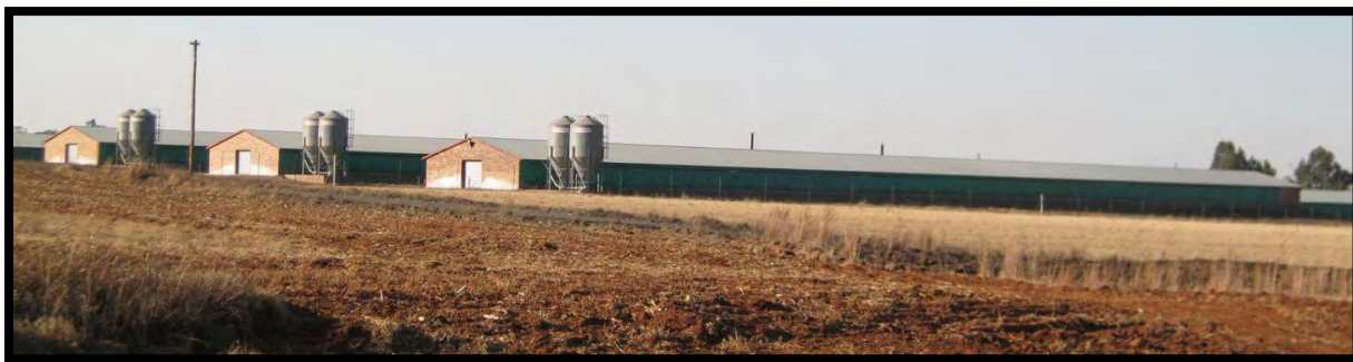
Figure 20: Brakchick infrastructure (number 12 in Figure 13)
