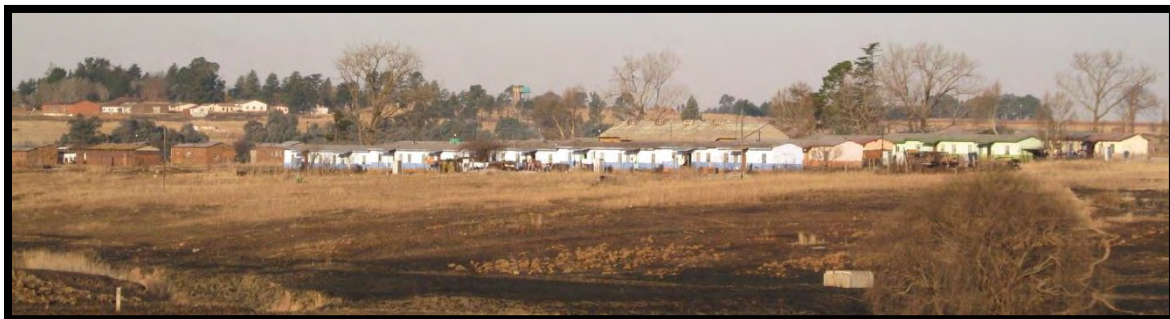
Figure 16: Mining compound (number 4 in Figure 13)
