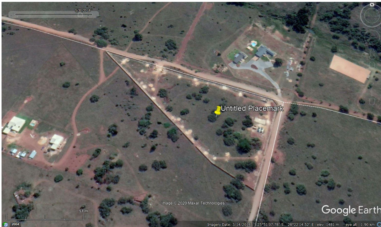
Figure 1-3: In 2017, the construction of the boundary wall commenced and was completed by April 2018. The construction of the staff accommodation and the pump room with the four JoJo tanks commenced in March 2018 and was completed in September 2018.
