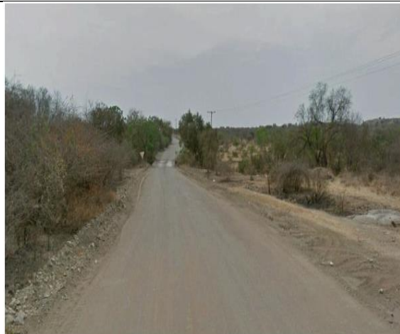
Figure 72: Access road (low-water bridge) just north of D2170
