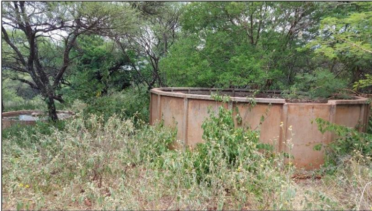
Figure 51: Cement dam at Site F09.
