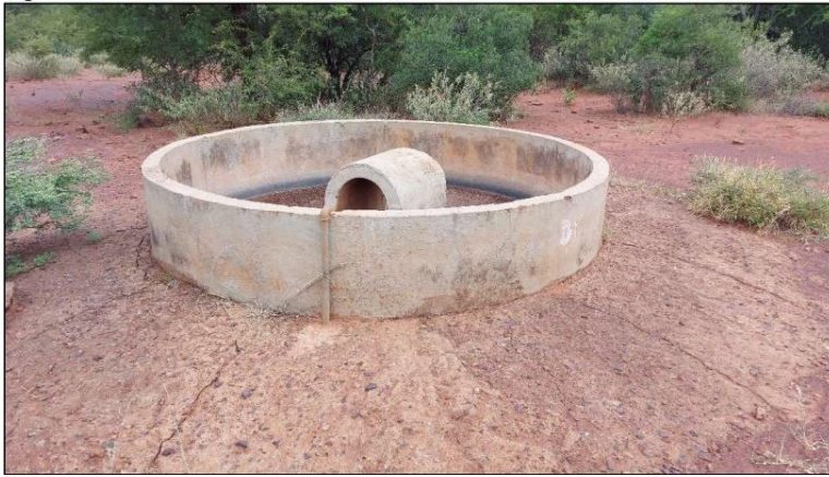
Figure 50: Cement dam at Site F08.
