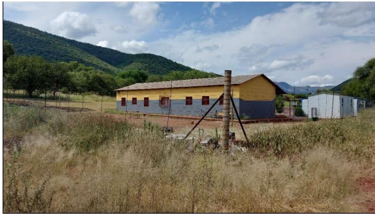
Figure 47: School at Site B04.
