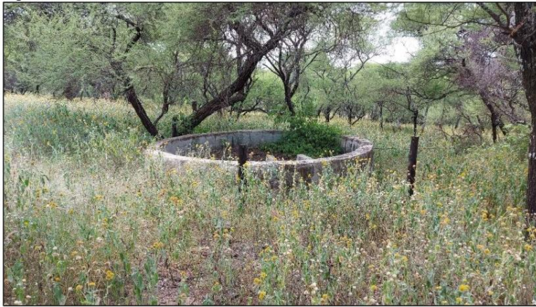
Figure 53: Small cement dam at Site B10.
