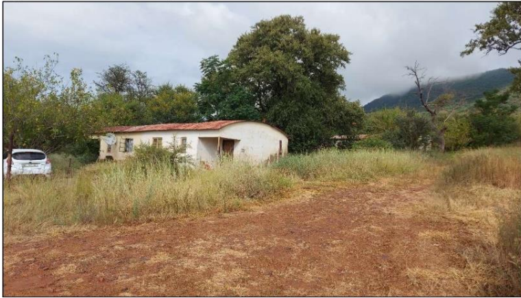
Figure 33: A remaining building at Site B03.
