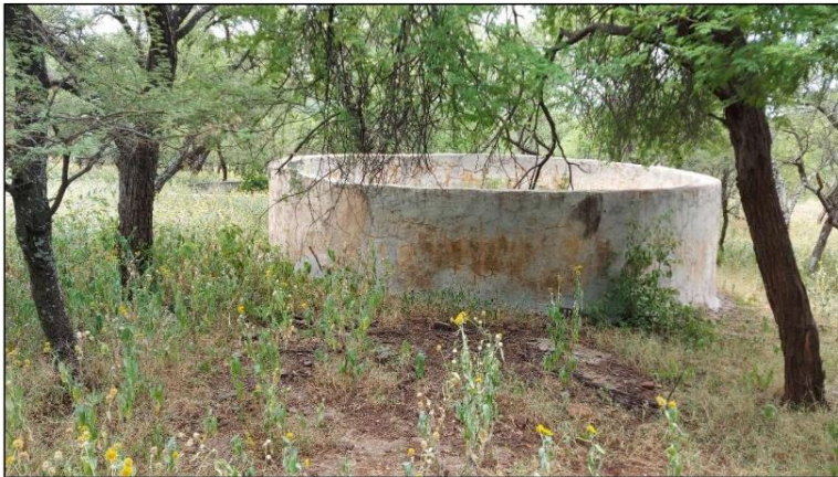
Figure 52: Cement dam at Site B10.
