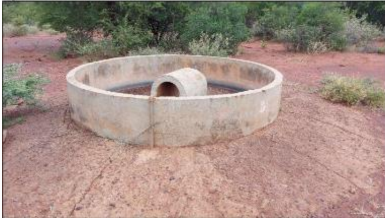
Figure 103: Cement dam at Site F08.
