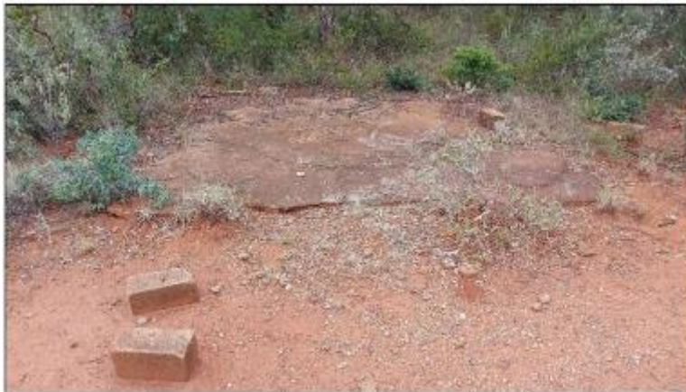
Figure 99: Building foundation / cement slab at Site F05.
