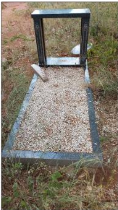
Figure 114: Broken surface feature at Cemetery B11.
