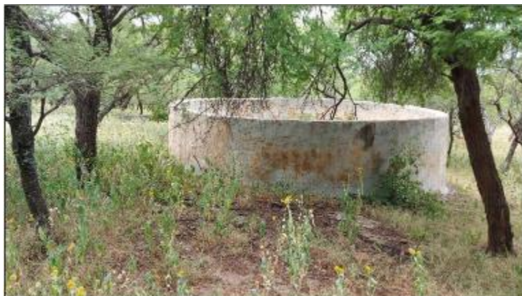
Figure 105: Cement dam at Site B10.
