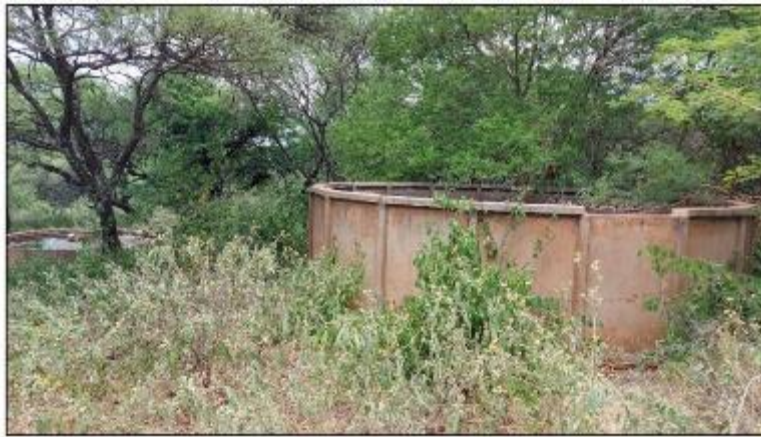
Figure 104: Cement dam at Site F09.
