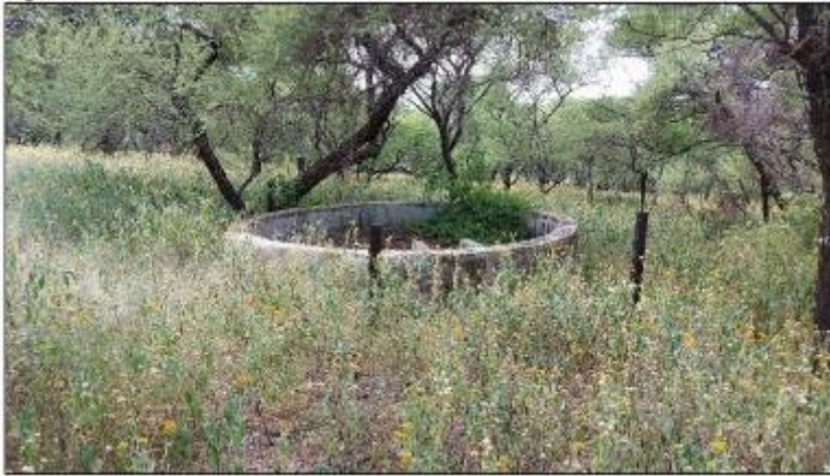
Figure 106: Small cement dam at Site B10.
