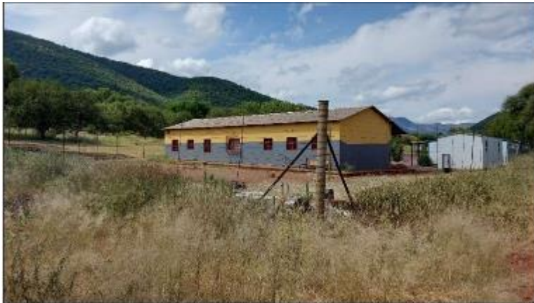
Figure 100: School at Site B04.
