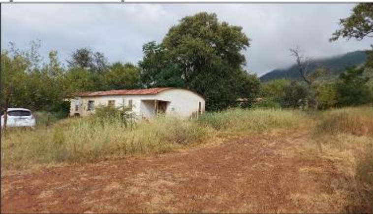
Figure 86: A remaining building at Site B03.
