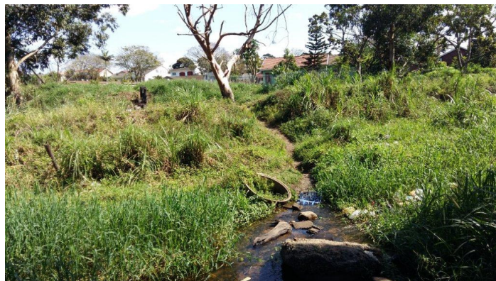
Plate 3 : Approx. alignment of crossing, looking west
