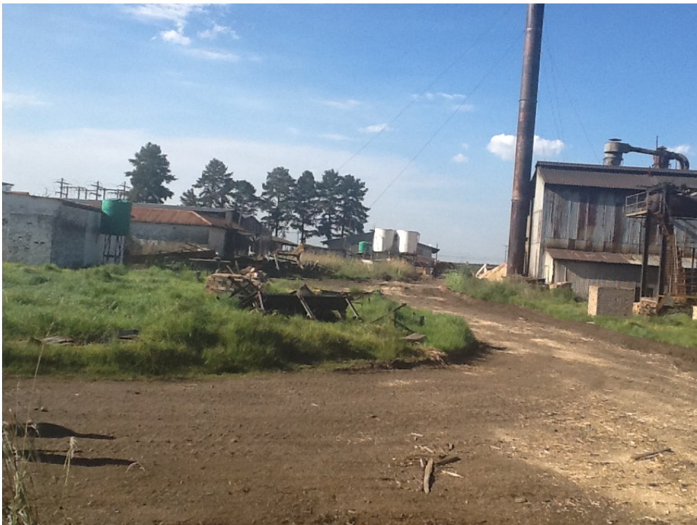
Figure 2: Area North from the existing boiler, where the new facilities will be erected
