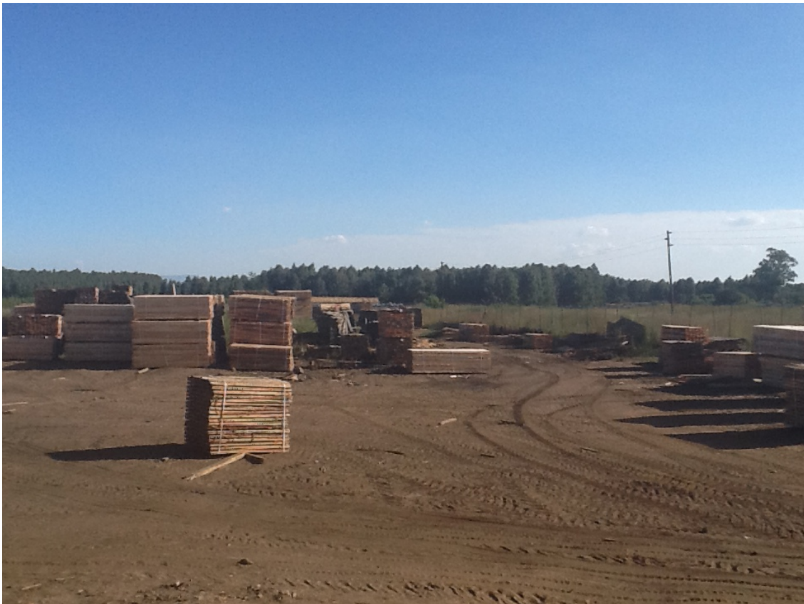
Figure 6: Area South West from the existing boiler, where the new facilities will be erected
