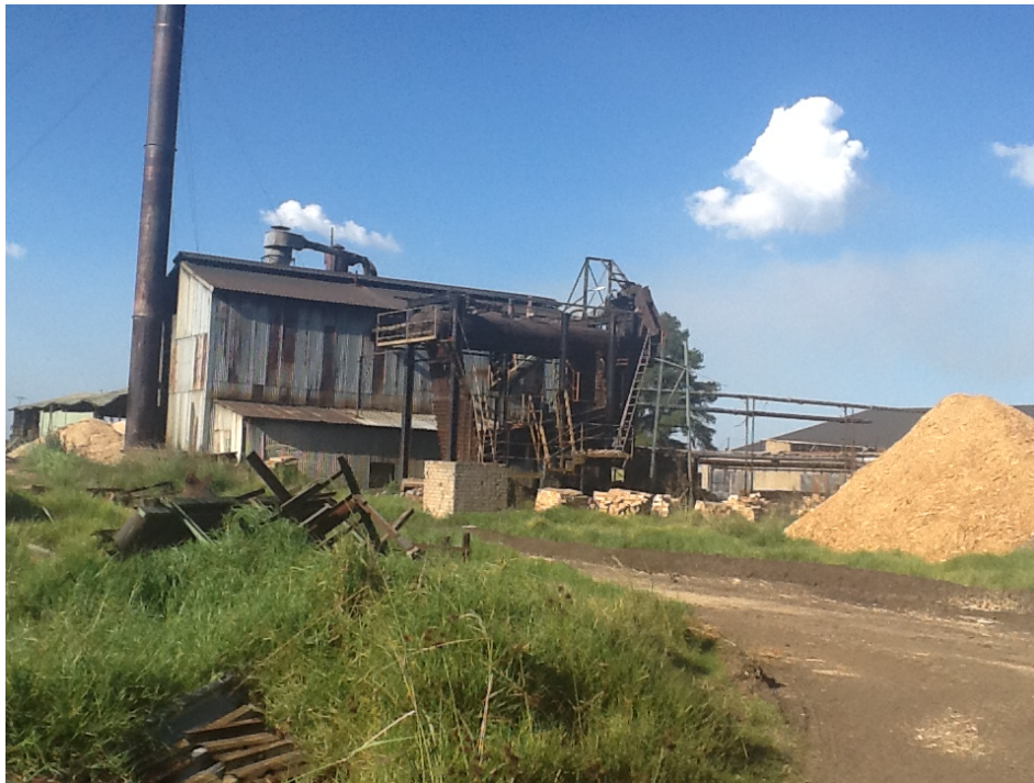
Figure 9: The old boiler house, which will be demolished.
