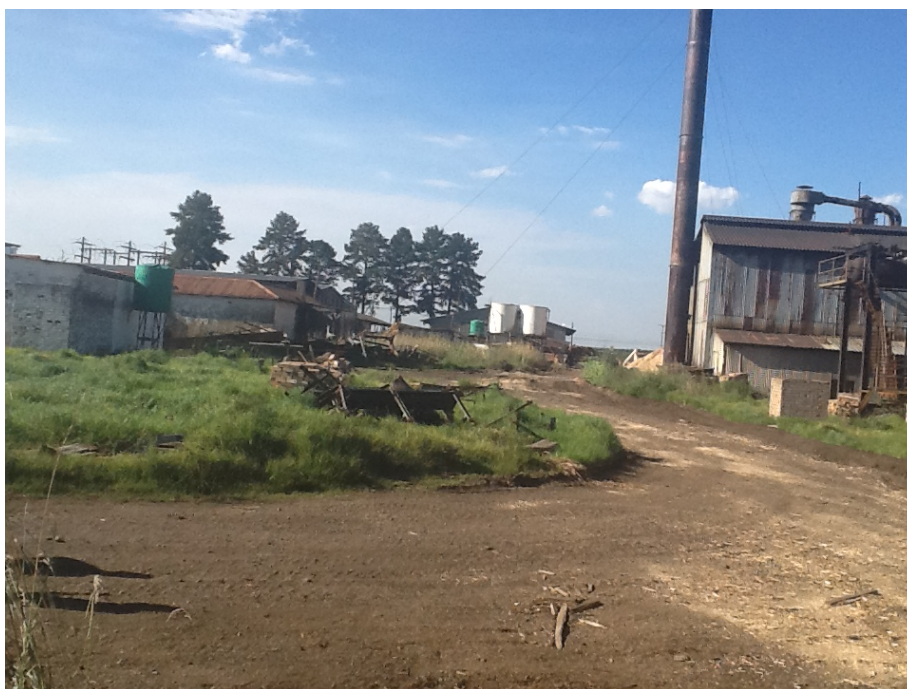
Figure 8: An overview of the site (with the existing boiler house to the right)
