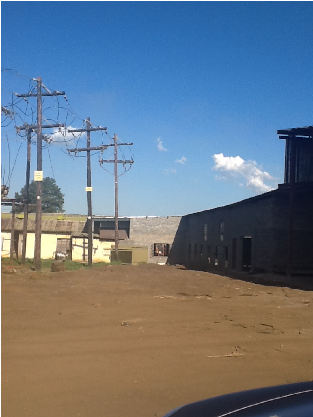
Figure 13: The current electricity distribution infrastructure on site, where the connection to the grid will be established
