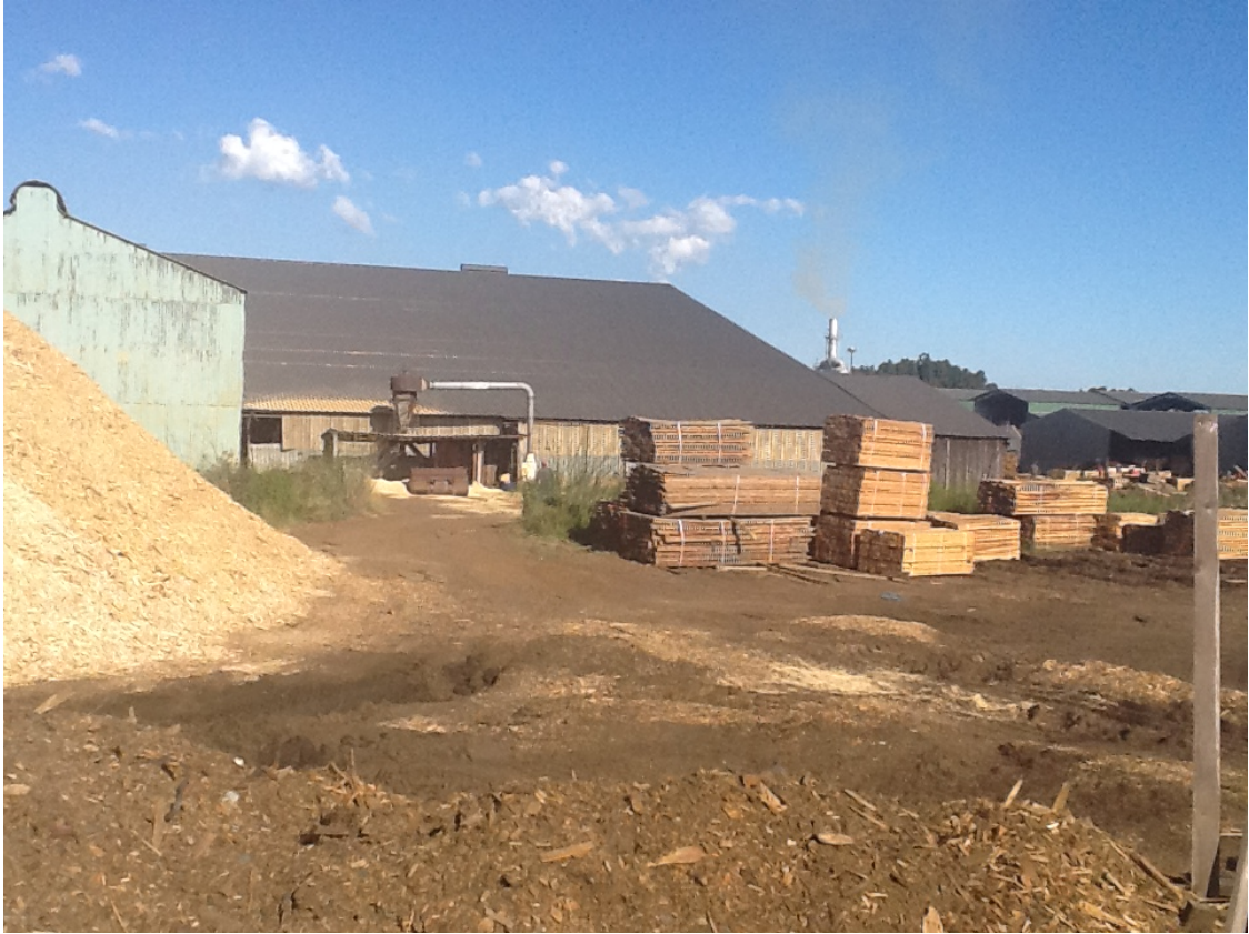
Figure 5: Area North East from the existing boiler, where the new facilities will be erected
