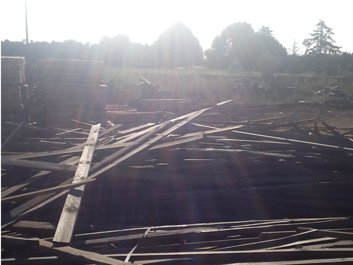
Figure 7: Area West from the existing boiler, where the new facilities will be developed
