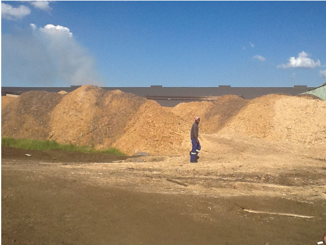
Figure 3 : Area East from the existing boiler, where the new facilities will be erected
