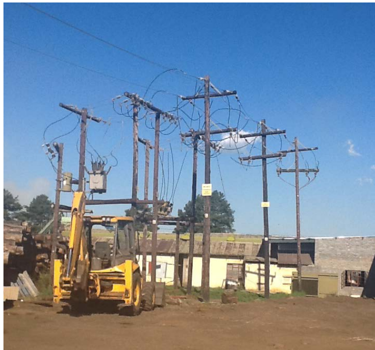
Figure 10: The existing electricity connection on the site, which will be used as the connection point for the generated electricity
