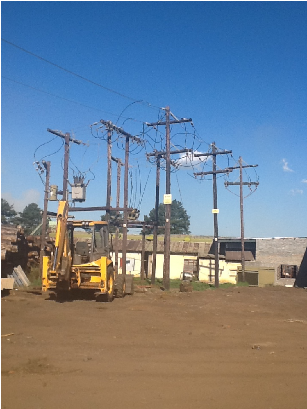
Figure 12: The current electricity distribution infrastructure on site, where the connection to the grid will be established
