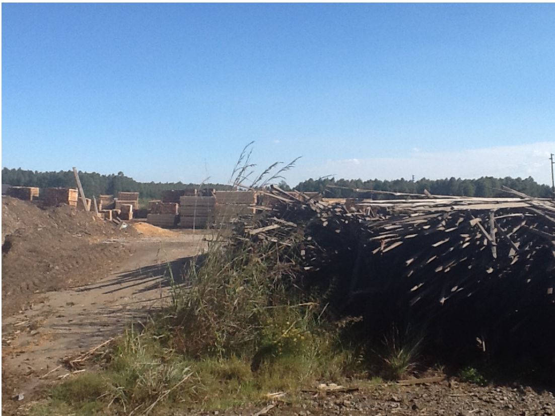
Figure 4: Area West from the existing boiler, where the new facilities will be erected
