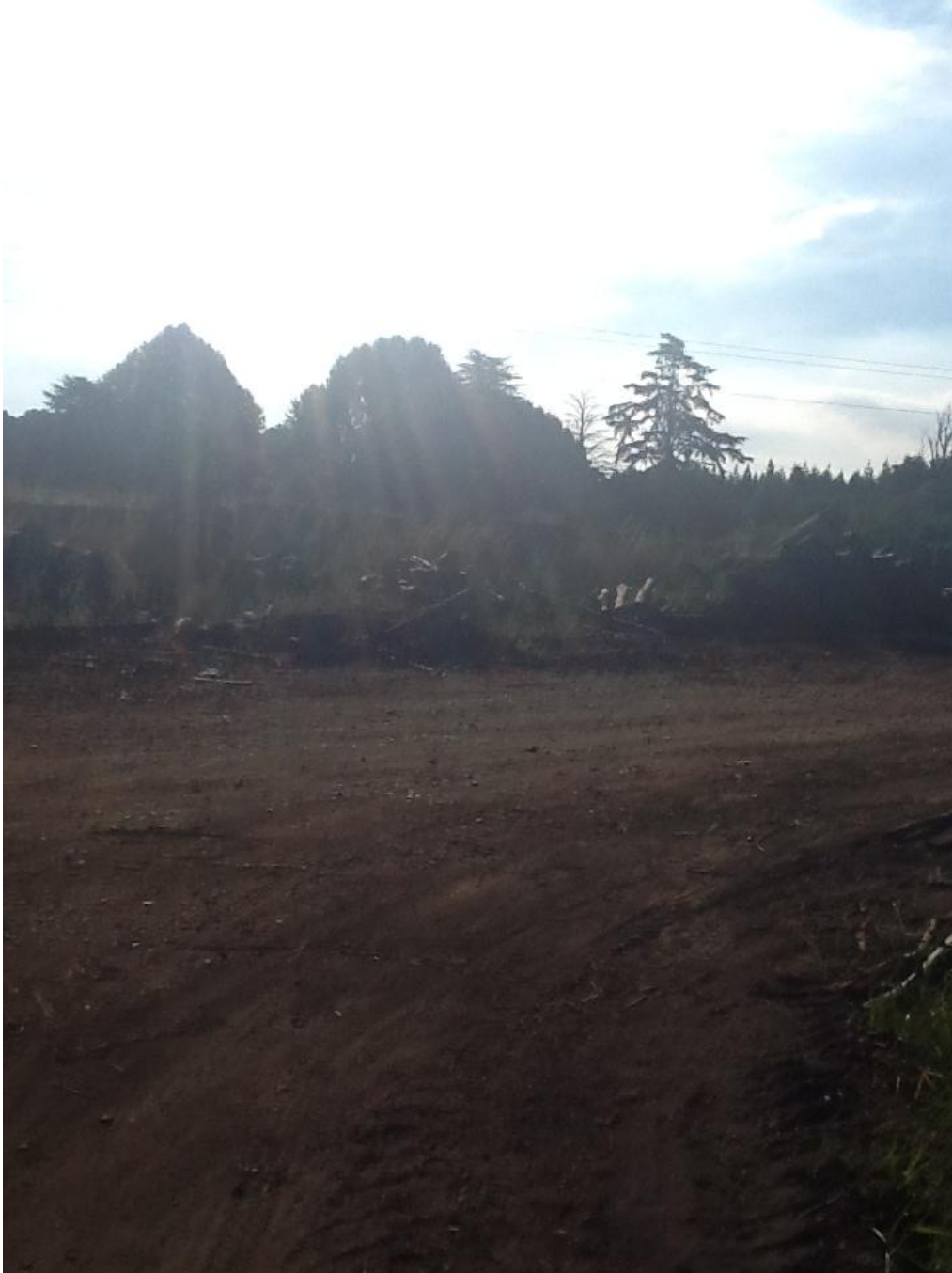
Figure 10: Area West from the existing boiler, where the new facilities will be developed
