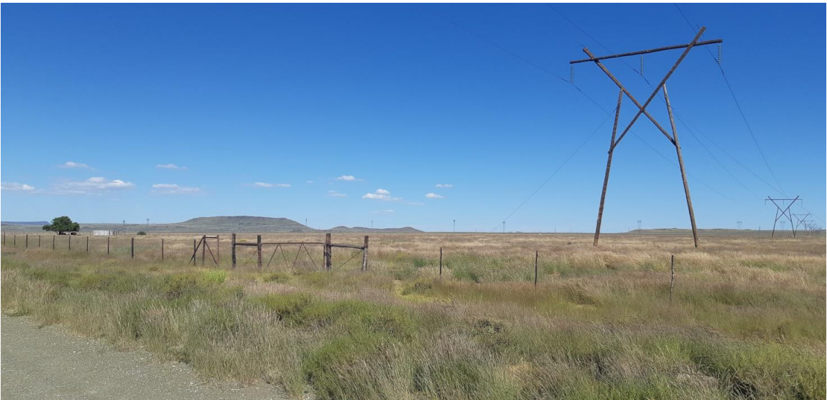
Looking south-east over the proposed Preferred Alternative power line route
