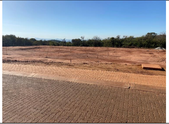
Construction camp for reservoir has been rehabilitated
