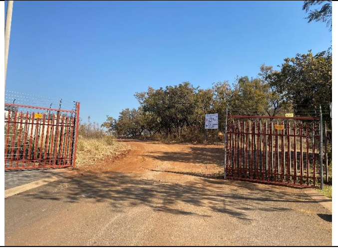
Entrance from Krokodilrivier (Rockridge Estate)
