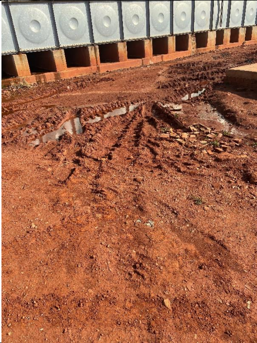
Water leaking from the RLM reservoir
