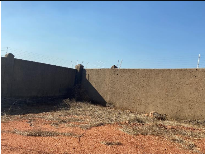
Existing boundary wall on North Western boundary
