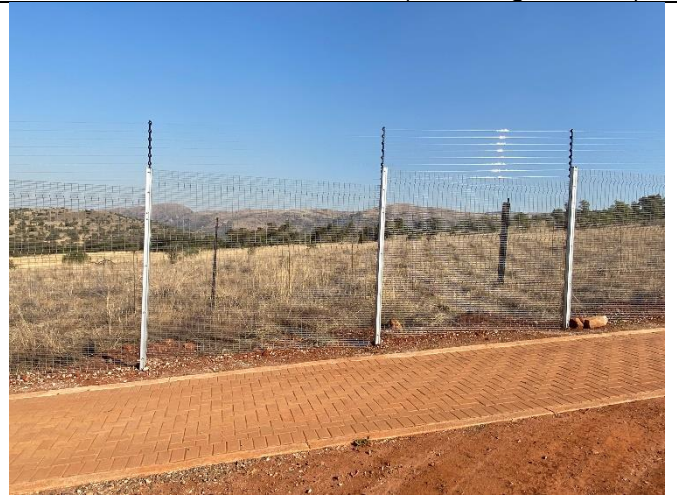
Old fence replaced with new fence due to security problems (Kgaswane boundary). Paved boundary road for patrolling – existing road that was paved.
