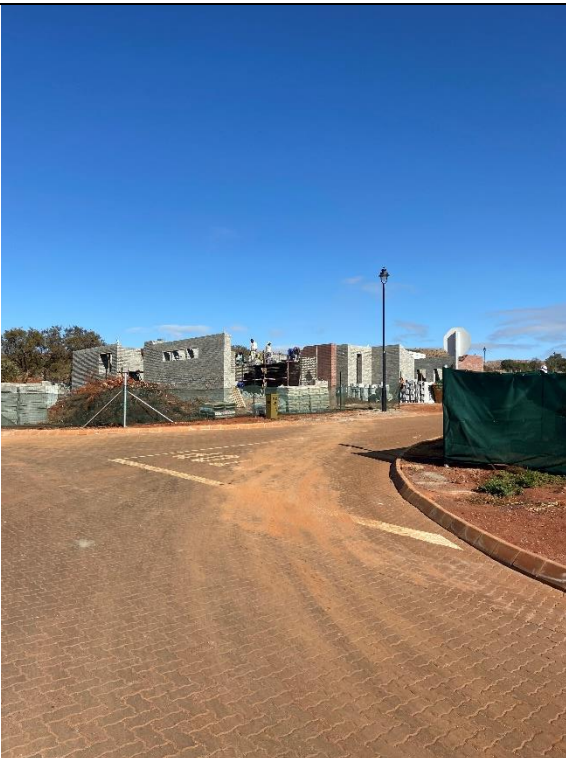
House being built in approved development area
